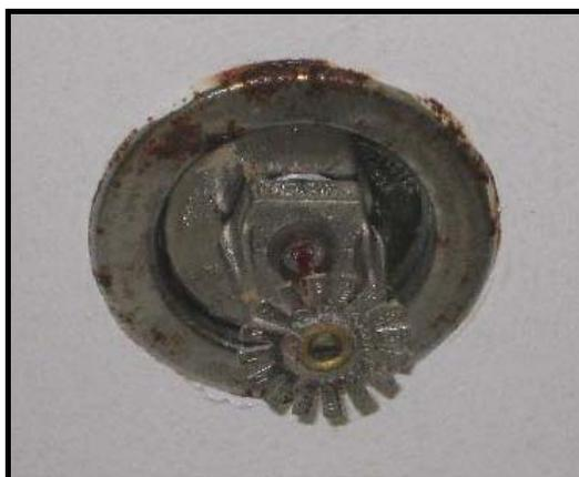
**Figure 3 – Corroded Sprinkler Escutcheon Plate**
