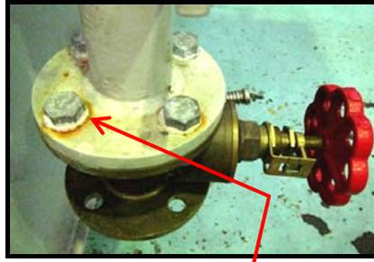
**Figure 4 – Corroded Bolts**
