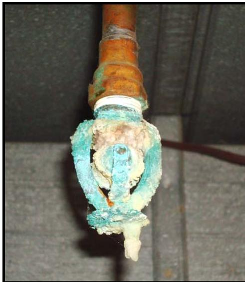
**Figure 2 – Corroded Sprinkler**
