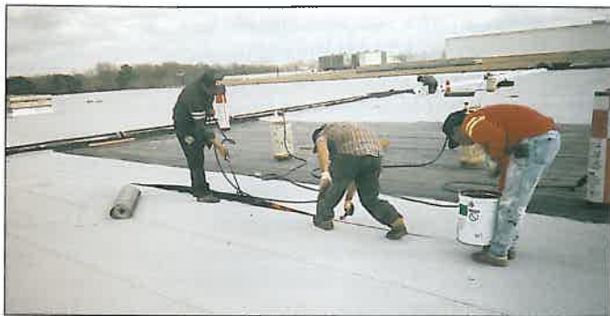
Fusing the side laps of a torch-applied modified bitumen cap sheet utilizing hand-held torching equipment, rolling the heated seam and embedding granules into the bleed-out.
