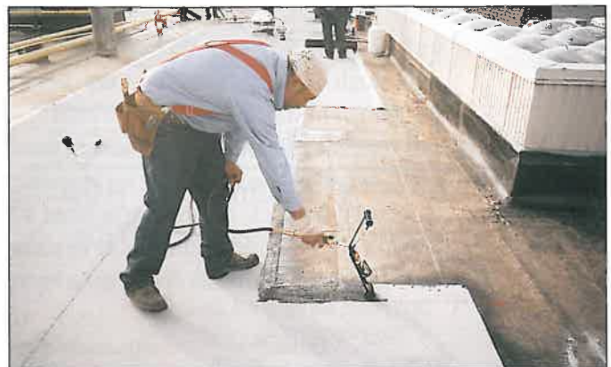
Installer heating granule surfacing at end lap of bottom sheet prior to applying overlying sheet.
