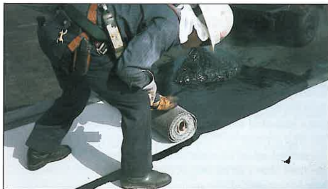
Installer applying downward pressure on cap sheet roll while maintaining roll in close proximity to asphalt mopping source.
