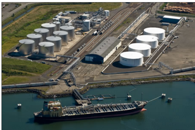
Terminal 1 at the Port of Grays Harbor operates as a barge and bulk liquid terminal. Photo courtesy of the Port of Grays Harbor.
