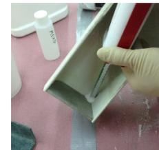
Use GutterGlue along edge of intersection between gutter & endcap. You can use your finger (with glove on) to smooth it out.
