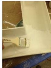
Use tongue depressor to wet out inside of seam with GutterGlue over fiberglass tape. Make sure to cover area so no fiberglass is showing and there are no voids. Trim excess fiberglass with utility knife and add some more glue to finish the top of gutter (Front and Back)
