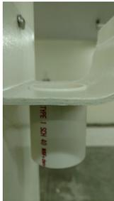
Outlet should be a tight fit to gutter. If it is loose or will not sit straight use 2P10 Superglue to hold it in place while applying final bonding agent.
