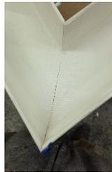
Wet out Fiberglass Tape with GutterGlue and lay into Miter/Seam.
