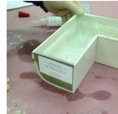
Stick Endcap in place so that it is flush with edge of gutter
