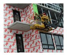
Knowing this, he selected 3M<sup>™</sup> Air and Vapor Barrier 3015 for the window flashing. 3M flashing accessories are extremely conformable and elongate in multiple directions, so you can get a good seal around corners and awkward shapes. They're also compatible with multiple substrates so you have fewer worries about sticking to all the materials that come together in one place.
