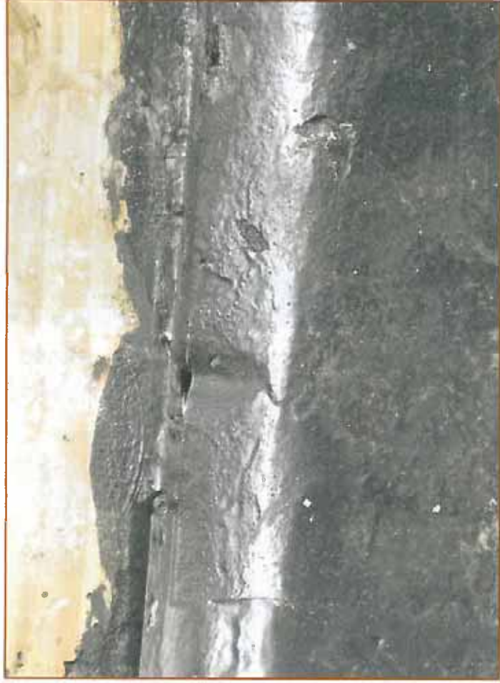
Photo 7 – Open fishmouth at top edge of felts.
