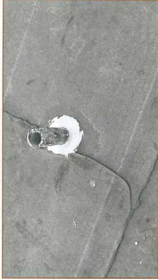
Photo 8 – Sealant applied around penetration on modified bitumen.
