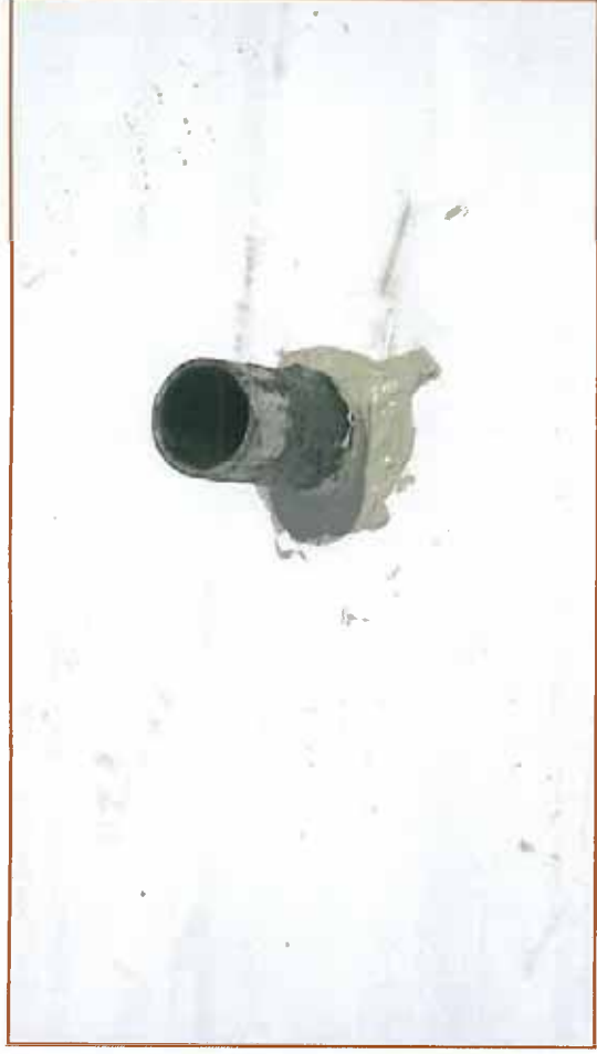
Photo 11 – Sealant applied around penetration in single ply as temporary seal.
