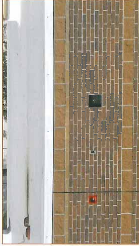
Photo 10 – Trimmed edge of single-ply at perimeter.
