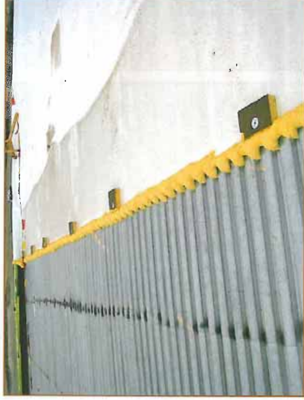
Photo 12 – Spray foam applied along tie-in of single ply on metal deck.
