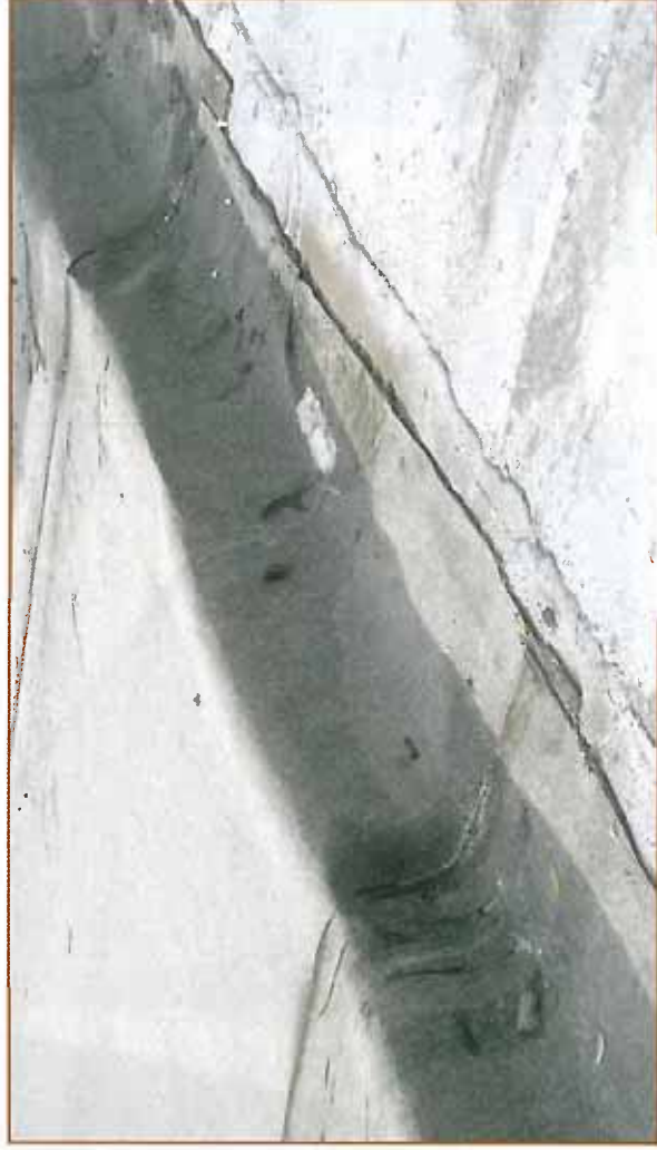
Photo 3 – Tie-in at deck.
