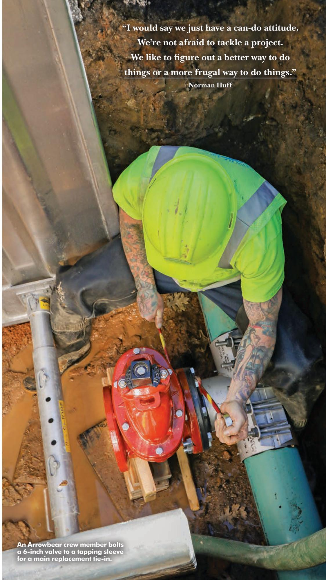
**An Arrowbear crew member bolts a 6-inch valve to a tapping sleeve for a main replacement tie-in.**
