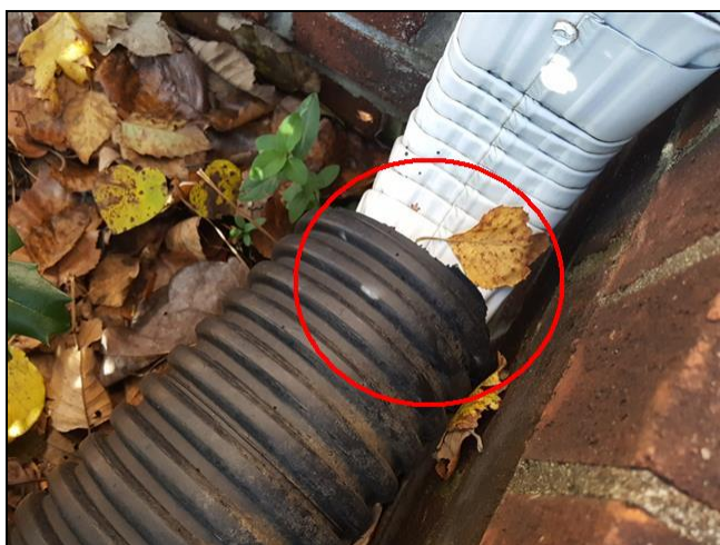
2.3 Item 10(Picture) front left corner of porch
