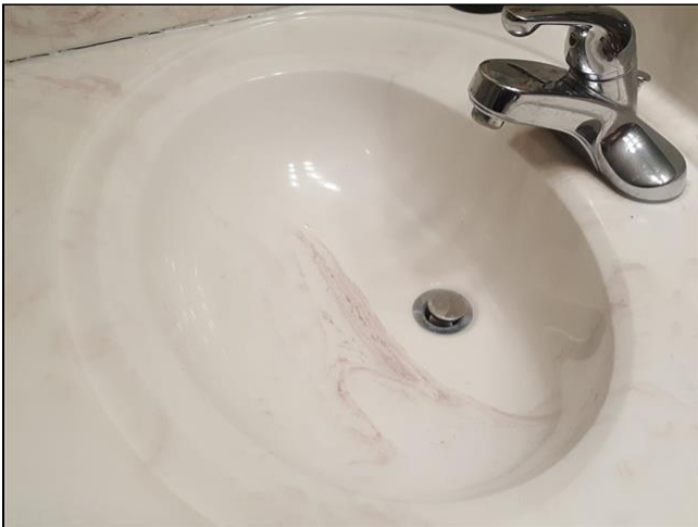
7.4 Item 1(Picture) master bathroom
