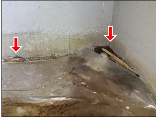
1.3 Item 2(Picture) front right corner of home
