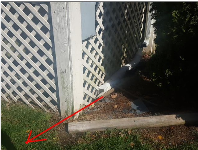
2.3 Item 4(Picture) rear right corner of patio porch
