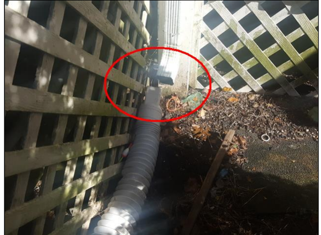
2.3 Item 11(Picture) rear right corner of patio porch
