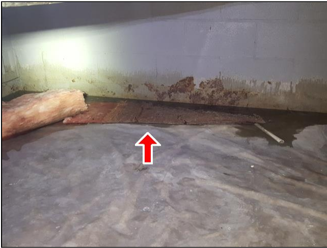
1.2 Item 7(Picture) front right corner of home
