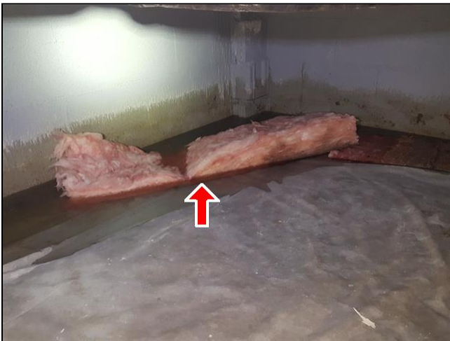
1.3 Item 3(Picture) under front entry
