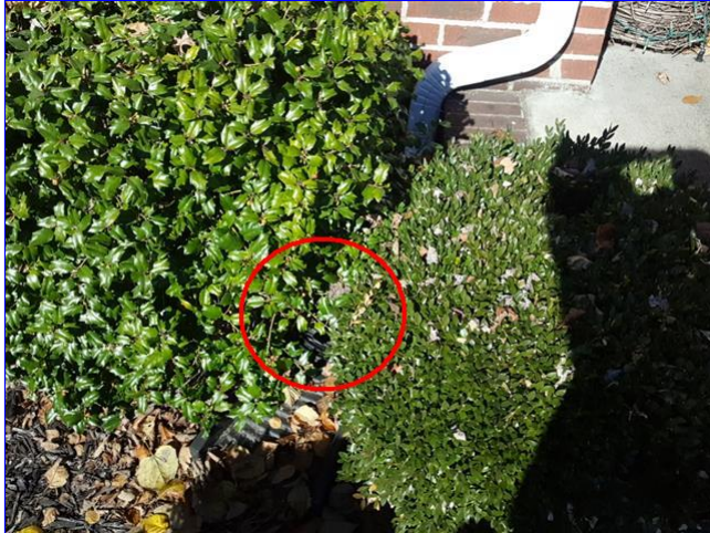
2.3 Item 8(Picture) front left corner of porch
