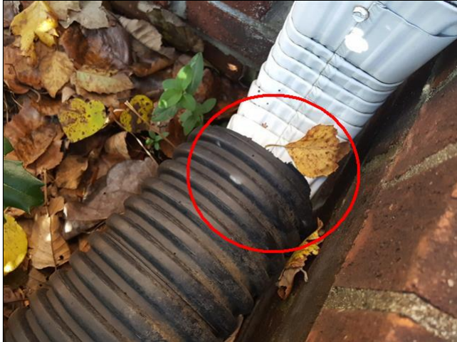
2.3 Item 10(Picture) front left corner of porch
