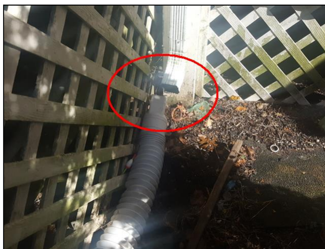
2.3 Item 11(Picture) rear right corner of patio porch
