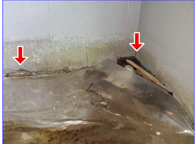
1.3 Item 2(Picture) front right corner of home
