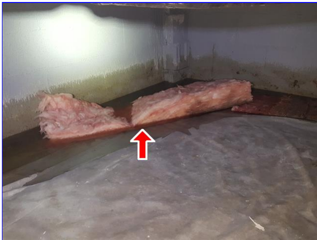
1.3 Item 3(Picture) under front entry
