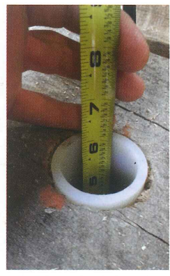
Pictured above are images of BTX ports. Left: A BTX port installed prior to injection. Center: A BTX port prior to capping filled with DOT borate (Cellutreat™). Right: A BTX port empty after the Boulton cycle using Copper Naphthenate.
