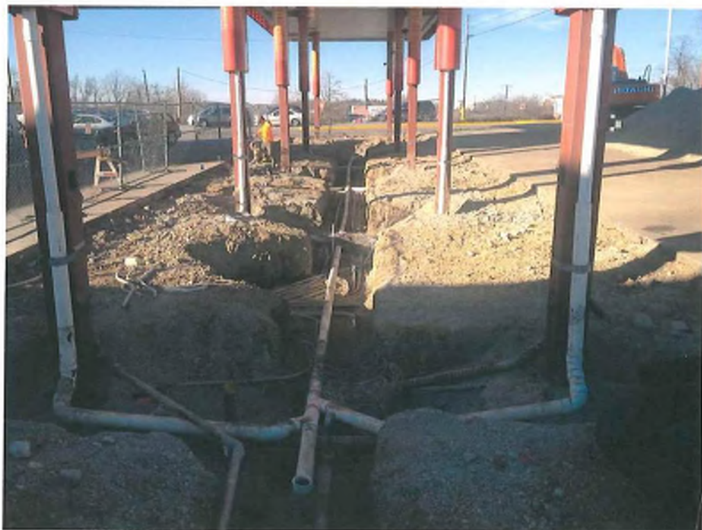
Pumps 1 through 10 after piping and sump removal
