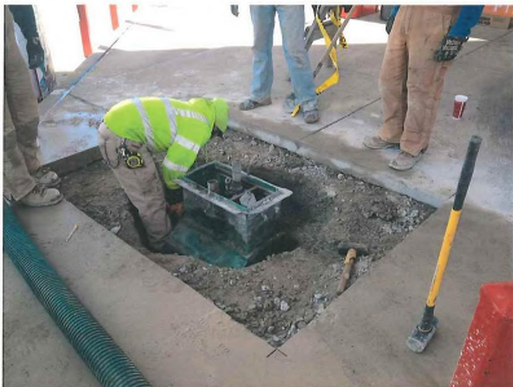
Excavation of kerosene sump
