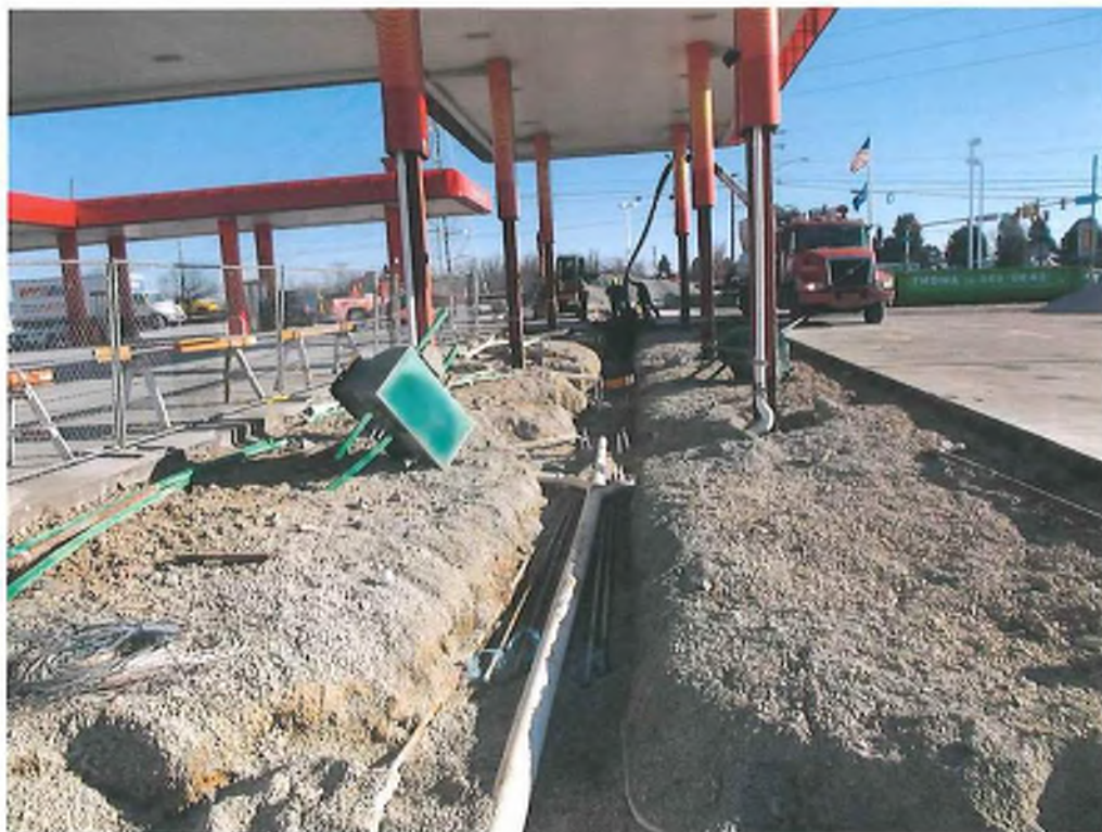
Pumps 11 through 18 after sump and piping removal, facing east/northeast
