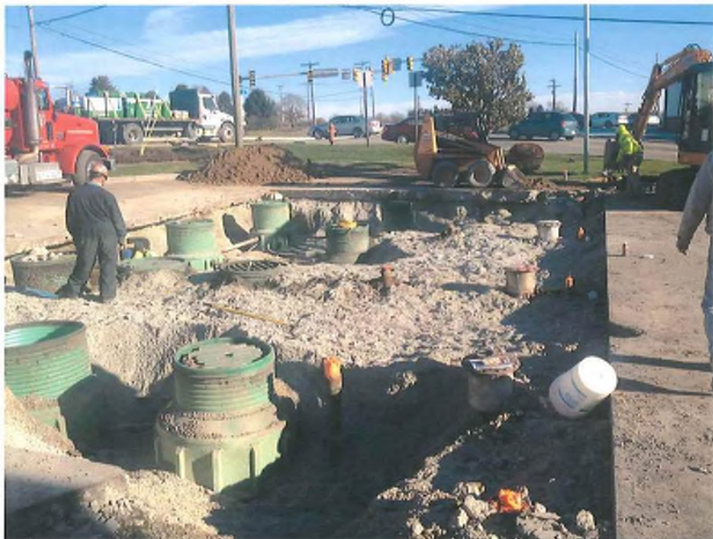
Tank top upgrades
