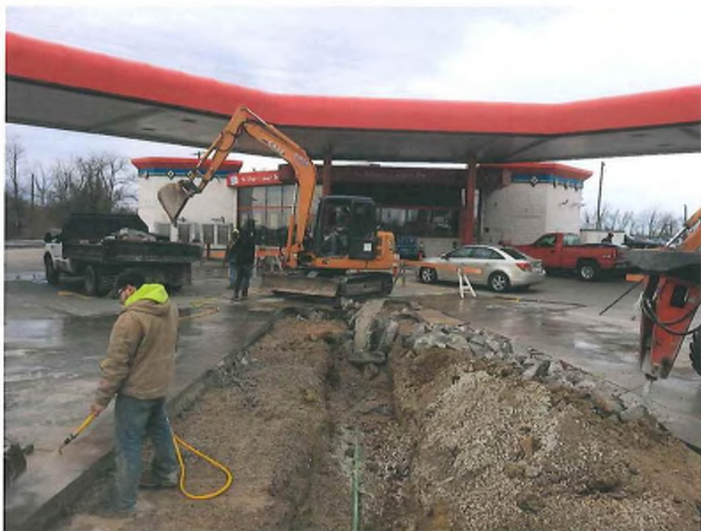
Kerosene line removal
