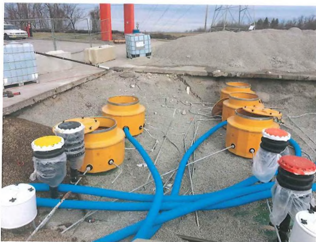
Tank top equipment
