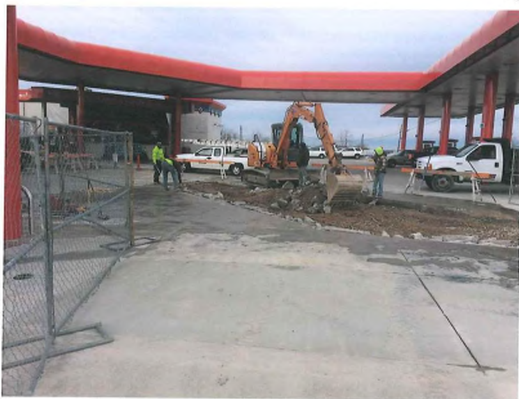
Kerosene line removal
