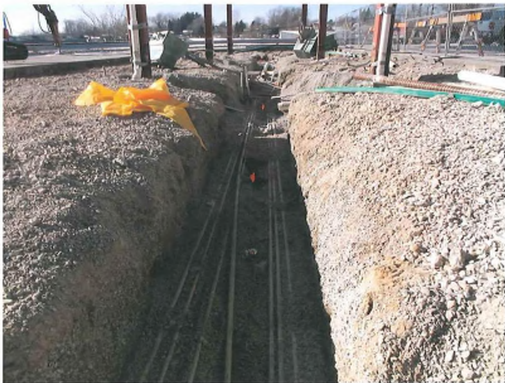
Product line trench with electrical conduits
