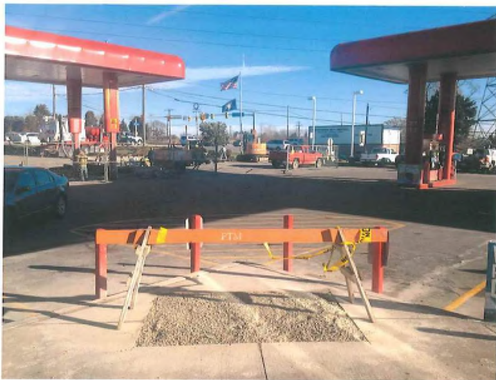
After removal of kerosene dispenser and sump, facing southeast
