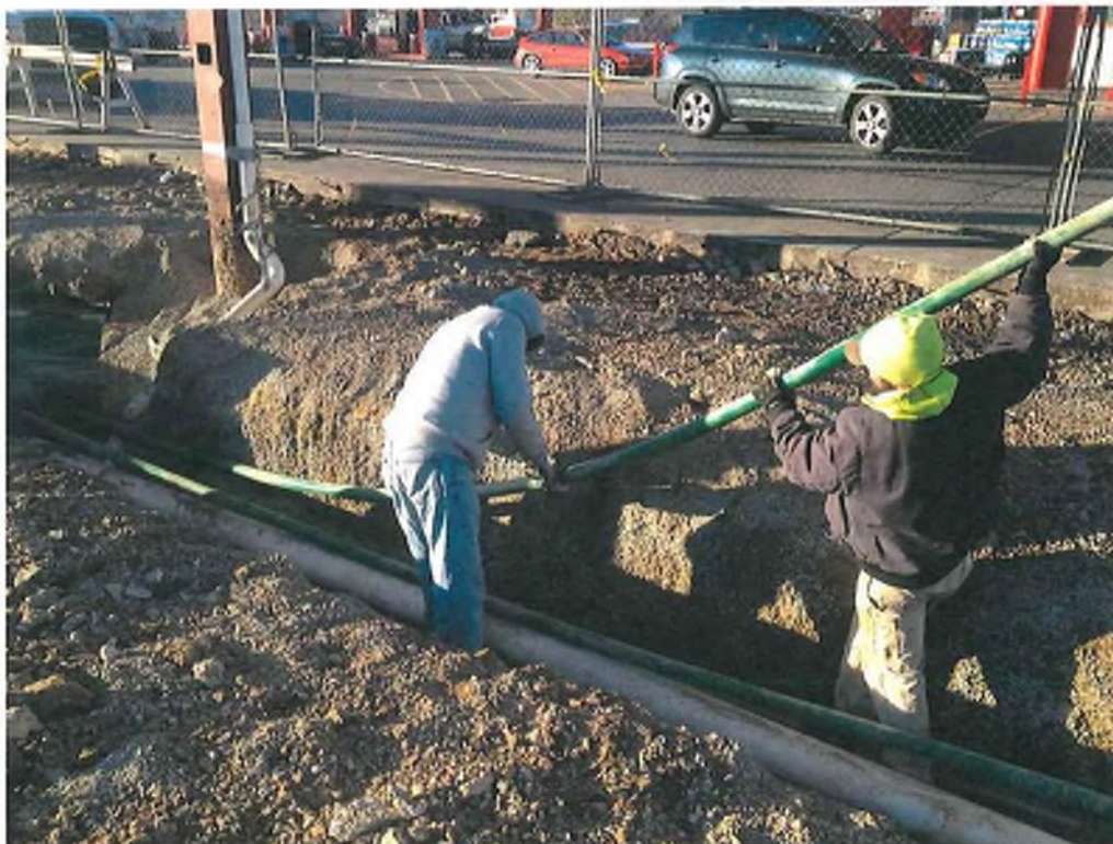
Removal of product piping at pumps 1 through 8
