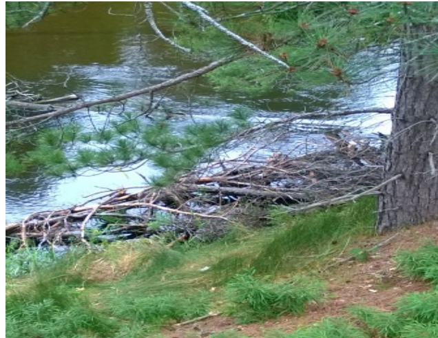
After: New structure, dense, great fish cover, improved bank stabilization
