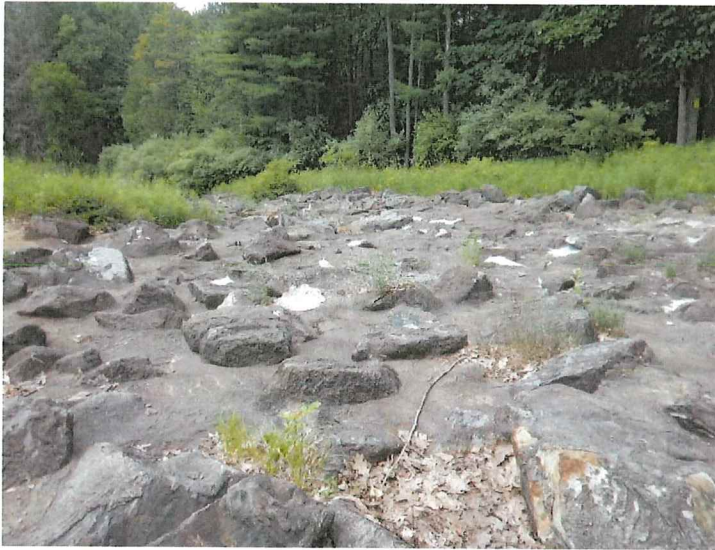
13. View looking downstream in the auxiliary spillway channel.
