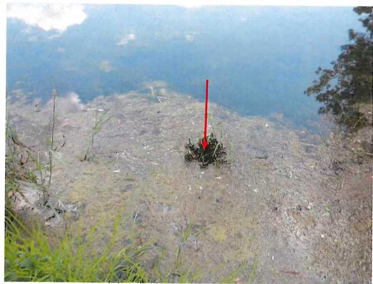
8. View of the principal spillway inlet.
