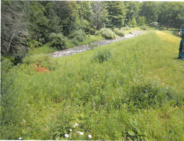
5. View of the downstream slope from the left abutment. Note the tall grass.
