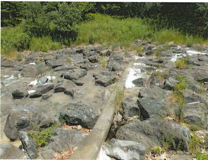
12. View of the concrete cut-off wall in the auxiliary spillway channel.
