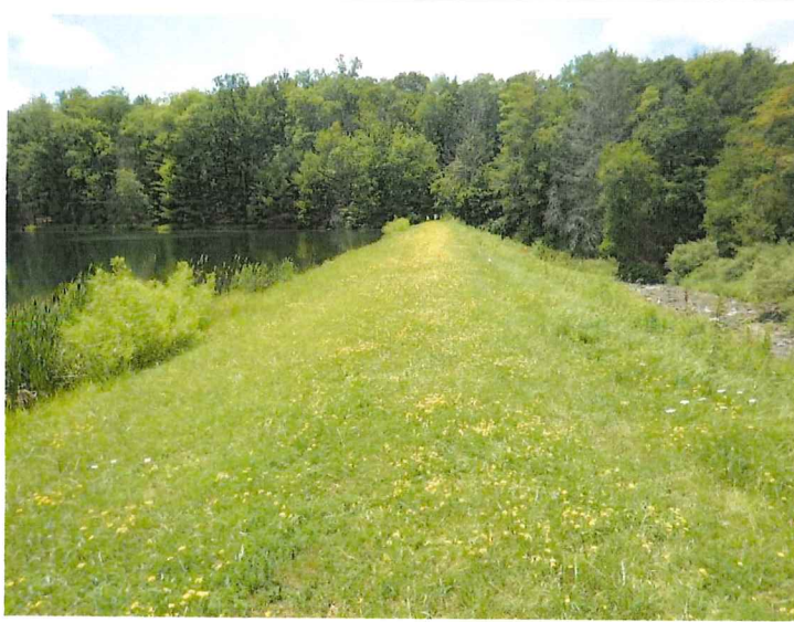
4. View of the crest of the dam from the right abutment.
