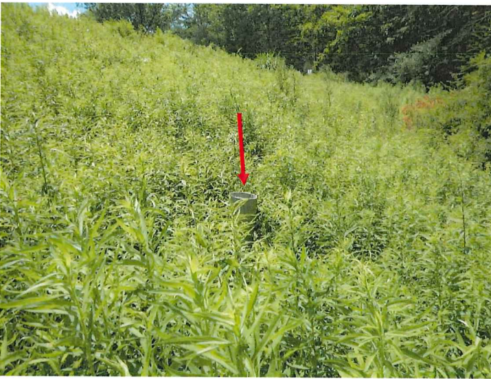
14. View of the lake drain valve control standpipe.
