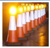
While drivers may get numb to seeing the same lane-closure warnings, the blinking cone lights seem to have caught their attention. During a typical night, workers often find that three or four of the reflective cones have been knocked over. However, none of the blinking lighted cones had been hit during the first few weeks of use.
