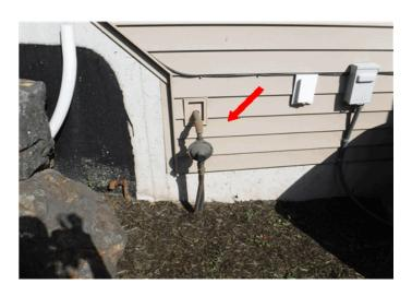
37) Gas Leak Check Inspected using Gas Trac NGX-6 Combustible Gas and Vapor
