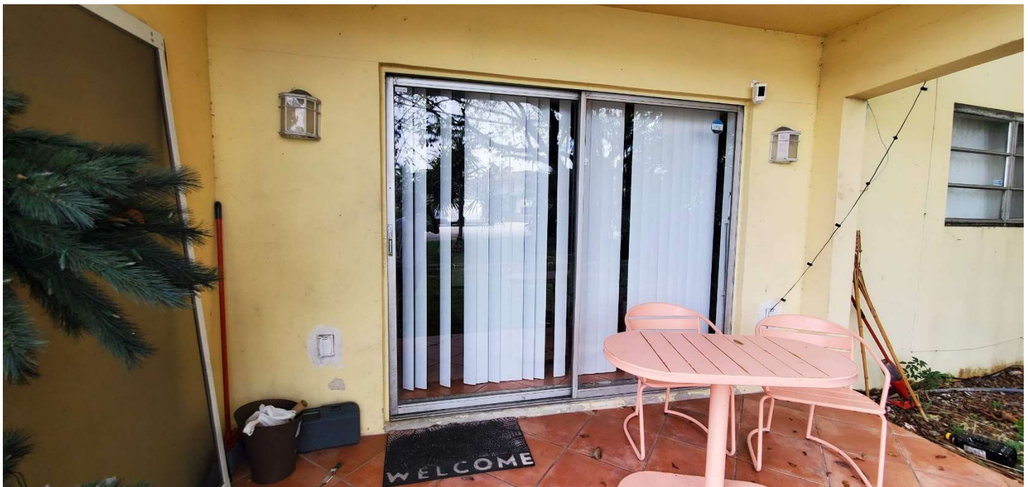
Sliding Glass Door, A 7300 AB 03 example of damaged door hardware allowing out of a plain moment of the door panel due to winds from Hurricane Irma.
