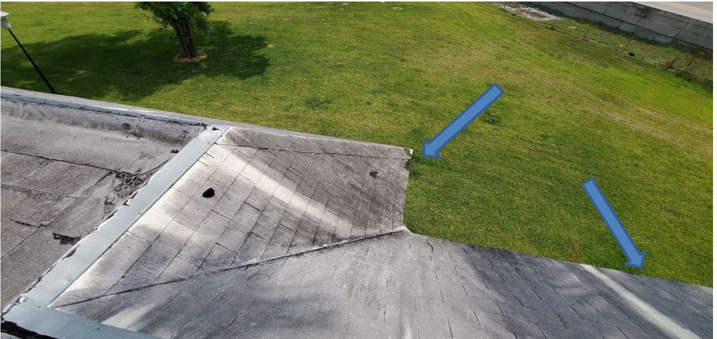
The roof of Building 7680; Example of wind damages to shingled mansards
