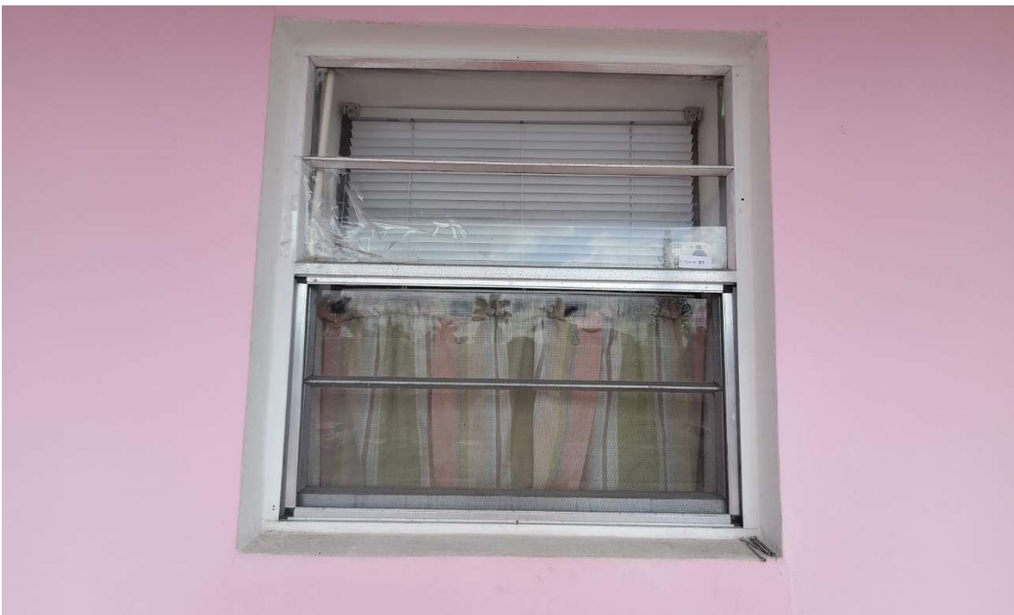
Single-hung window G-7500 BF-07 example of broken window glazing due to impacts from debris from Hurricane Irma
