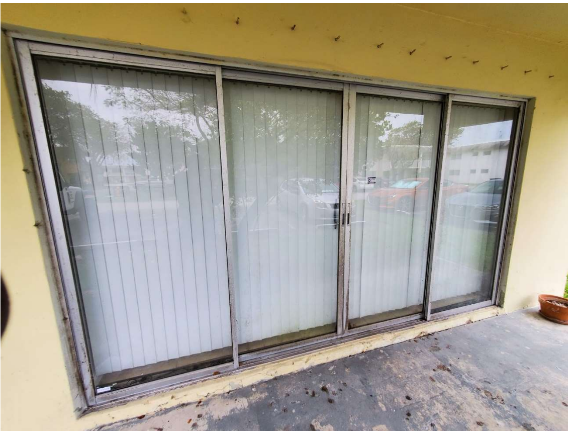
Sliding glass door, A-7310-AB-06 Example of the door without plane movement of the door panel.
