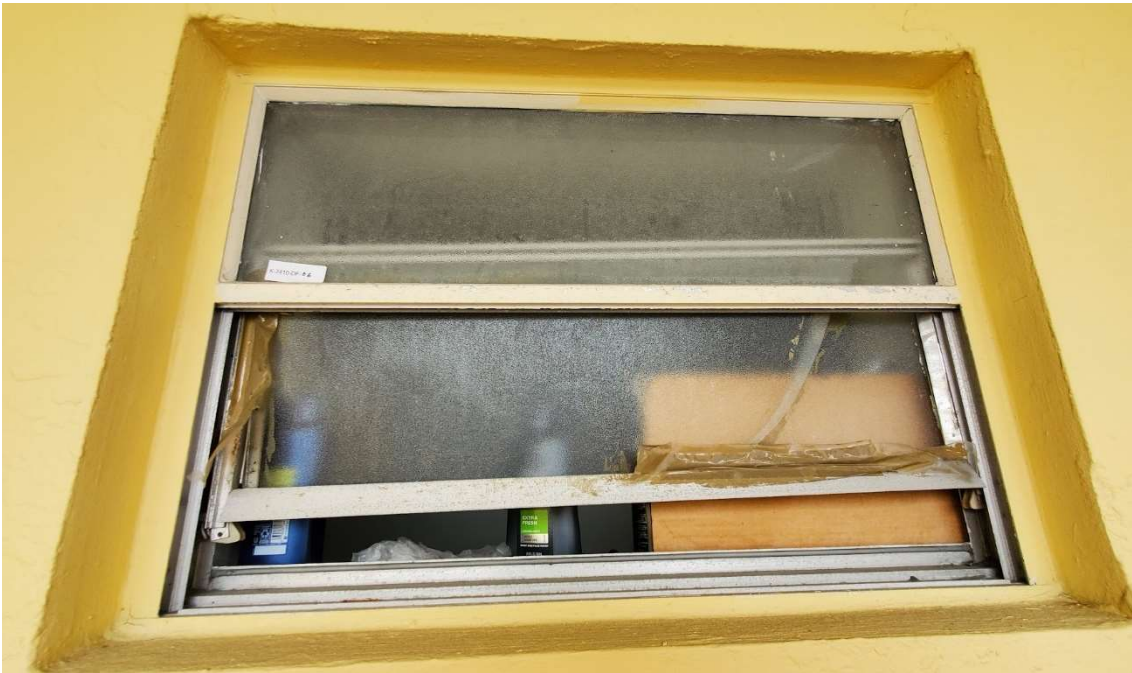
Single Hung Window K-7410-DF-06 example of a window with a damaged window sash, balancer, and cracked glass pane. These damages are a result of the window balancers being dislodged by the wind pressures and vibrations from Hurricane Irma causing binding and deformation of the sash.
