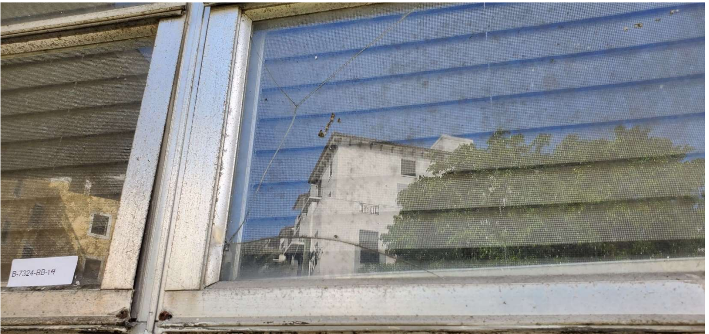
Window B-7324-BB-14 is another example of an owner who has attempted to screw the awning closed on the window and impact damage cracking the glazing of the window due to Hurricane Irma.
