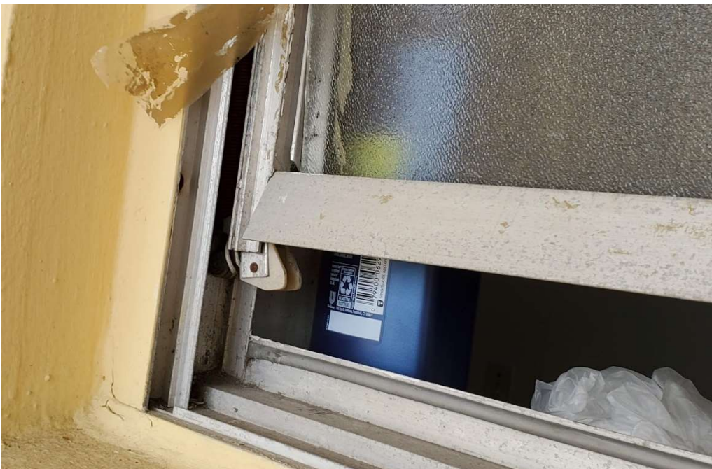
Single Hung Window K-7410-DF-06 example of a window with a damaged window sash, balancer and cracked glass pane. These damages are a result of the window balancers being dislodged by the wind pressures and vibrations from Hurricane Irma causing binding and deformation of the sash.
