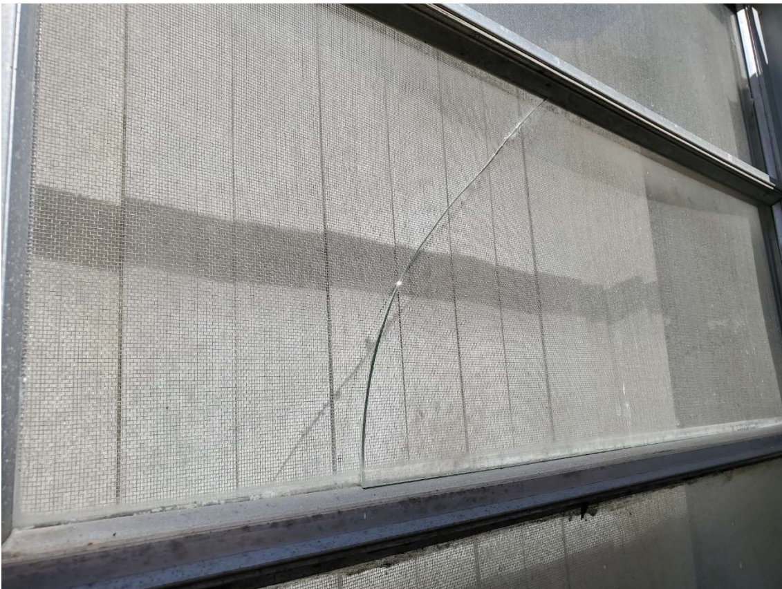
Awning Window C-7350 AL-01 example of broken window glazing due to deflection of the window awning frame.
