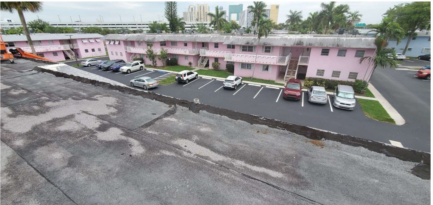
The roof of Building 7530; Example of delimitation of the build-up roof from the eave metal around the perimeter of the roof that has temporary repairs performed that were performed by the management company.
