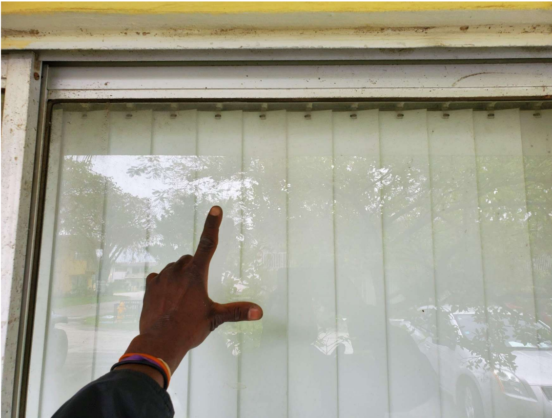
Sliding glass door, A-7310-AB-06 Example of the door without of plane movement of door pane. A photo with an L made with the fingers indicates that the door was inspected and exhibited out of the plane movement of the door panels.
