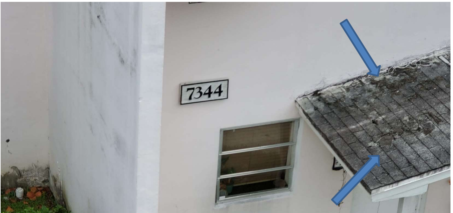
The roof of Building 7344; Example of wind damages to the shingled roof overhang
