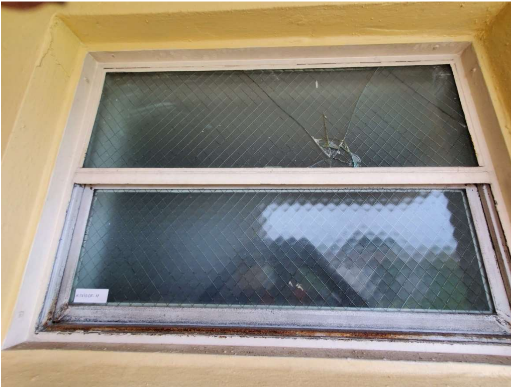
Single Hung Window K-7410-DF-11 example of a window with damage to broken glazing due to wind-borne debris from Hurricane Irma
