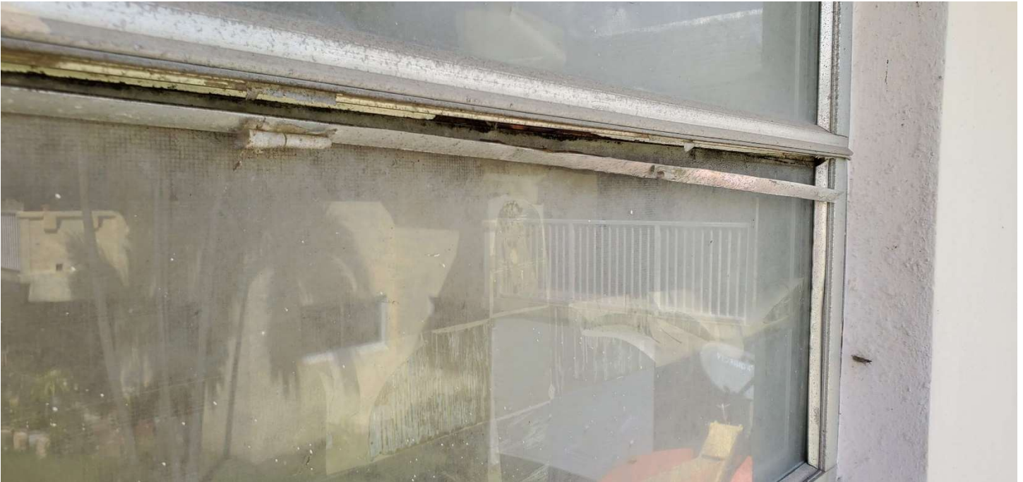
Awning Window B-7320-BR-04 Example of loose glazing due to negative wind pressures from Hurricane Irma
