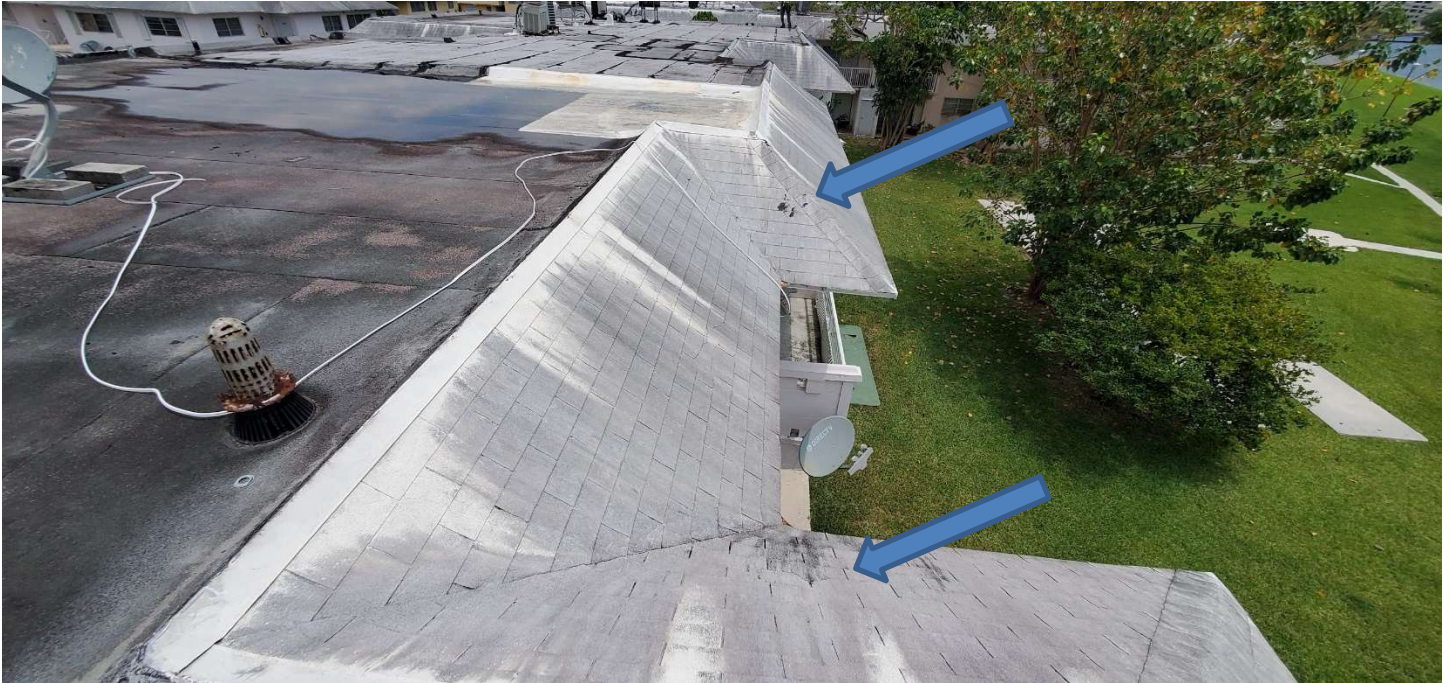
The roof of Building 7420; Example of wind damages to shingled mansards
