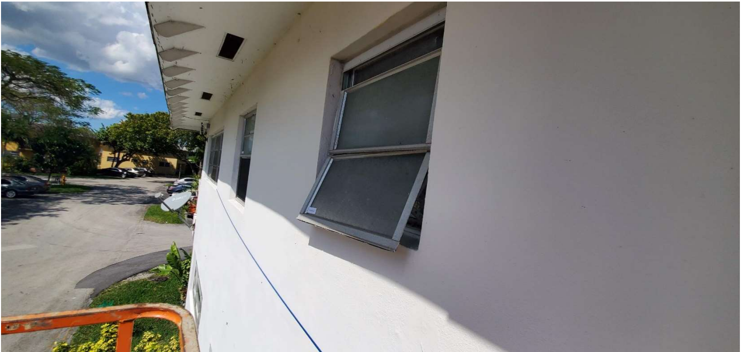
Awning Window B-7320-BL-03 Example of a loose window awning. The window awning locking mechanism and hardware have been damaged by the wind pressures from Hurricane Irma. Due to this damage, the window cannot close and is stuck in an open position.
