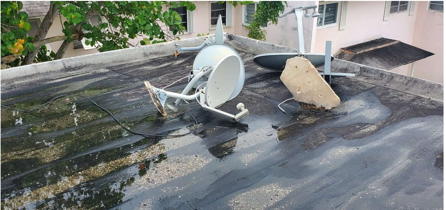
The roof of Building 7340; Example of wind-borne debris in the form of satellites that were blown around on the roof deck causing damage, there is also evidence of damages perlite roof insulation allowing water to pool on the roof deck.
