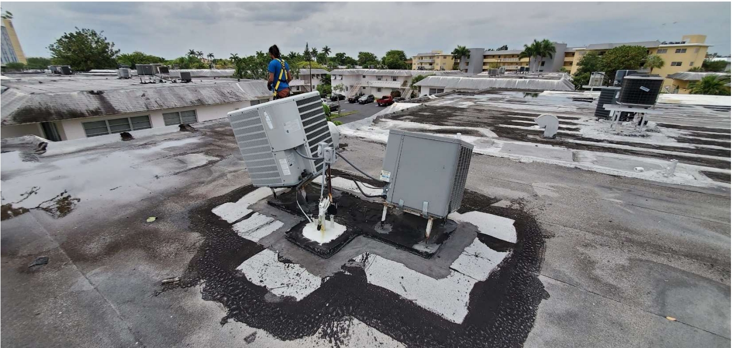
The roof of Building 7350; Example of damages to A/C condenser units and A/C stands on the roof, a temporary roof repair has been made around the stands to prevent further water intrusion.
