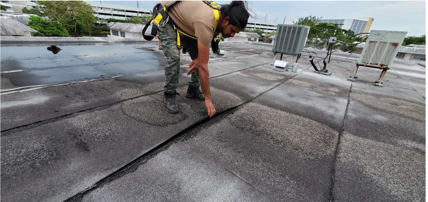
The roof of Building 1217; an example of up-lift pressures causing delamination of the “modified bitumen membrane” top ply at the seams of the roof and ponding water on the roof deck as a result of water damage perlite roof insulation collapsing.
