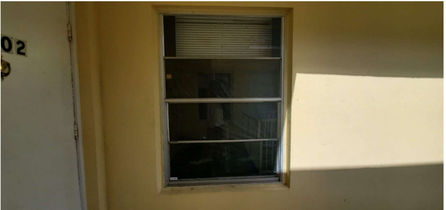
Single Hung Window A-7300-BF-05; Example of the single hung window that has new temporary glazing installed due to the original glass being broken from Hurricane Irma.
