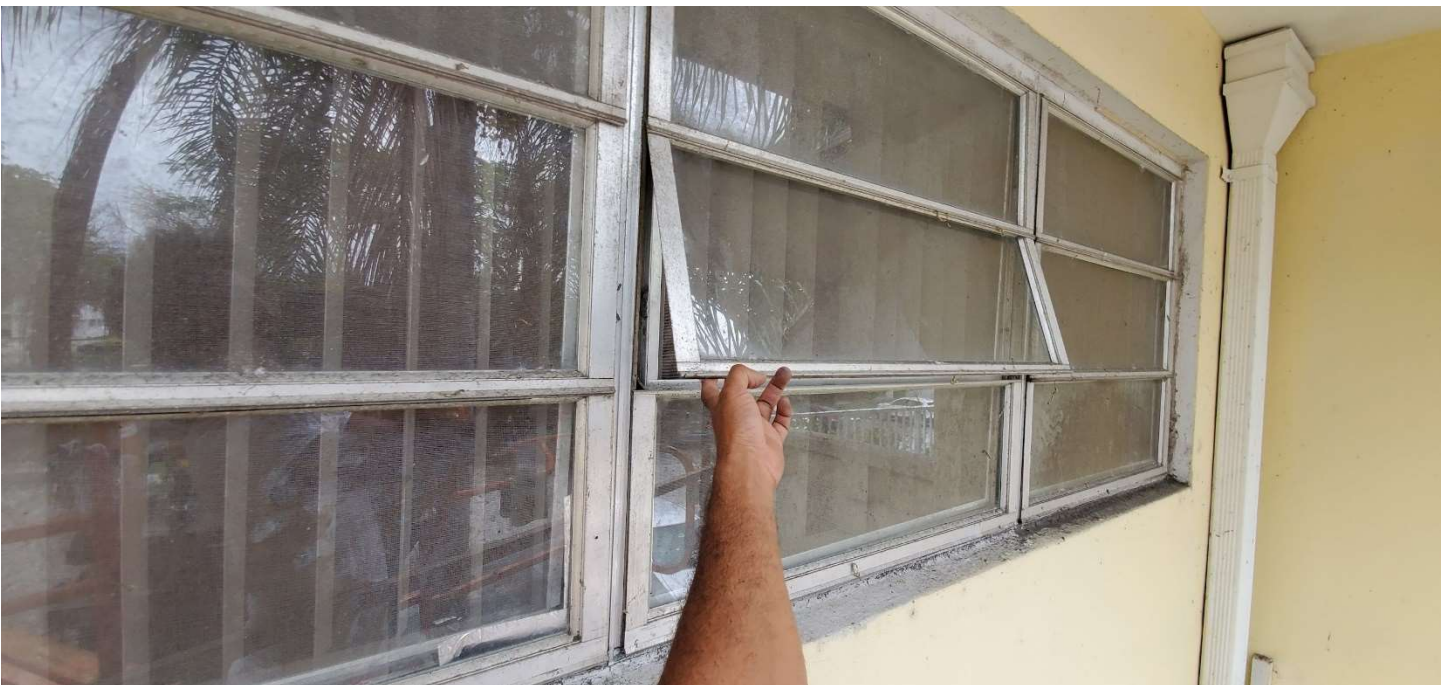
Awning Window A-7310-BB-05 Example of a loose window awning. The window awning locking mechanism has been compromised by the wind pressures from Hurricane Irma. Due to this damage, the window cannot be locked or be weather tight.
