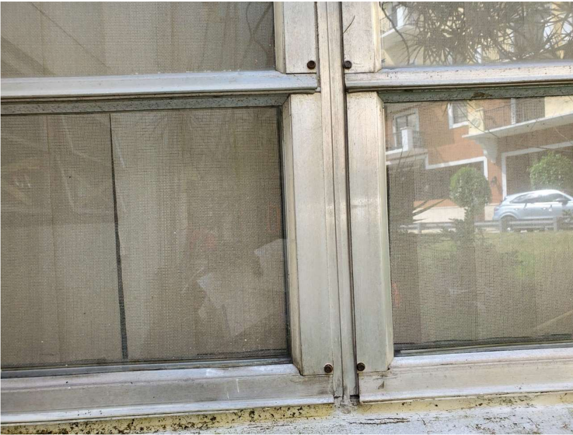
Awning Window B-7324-AB-05 this window has been screwed closed with self-taping screws from the outside by the owner to keep the window closed and attempt to make the window weather tight. This is another example of winding/ locking mechanisms being affected by the wind pressures from Hurricane Irma. Without the screws installed by the owner, the window would flap or sag open.
