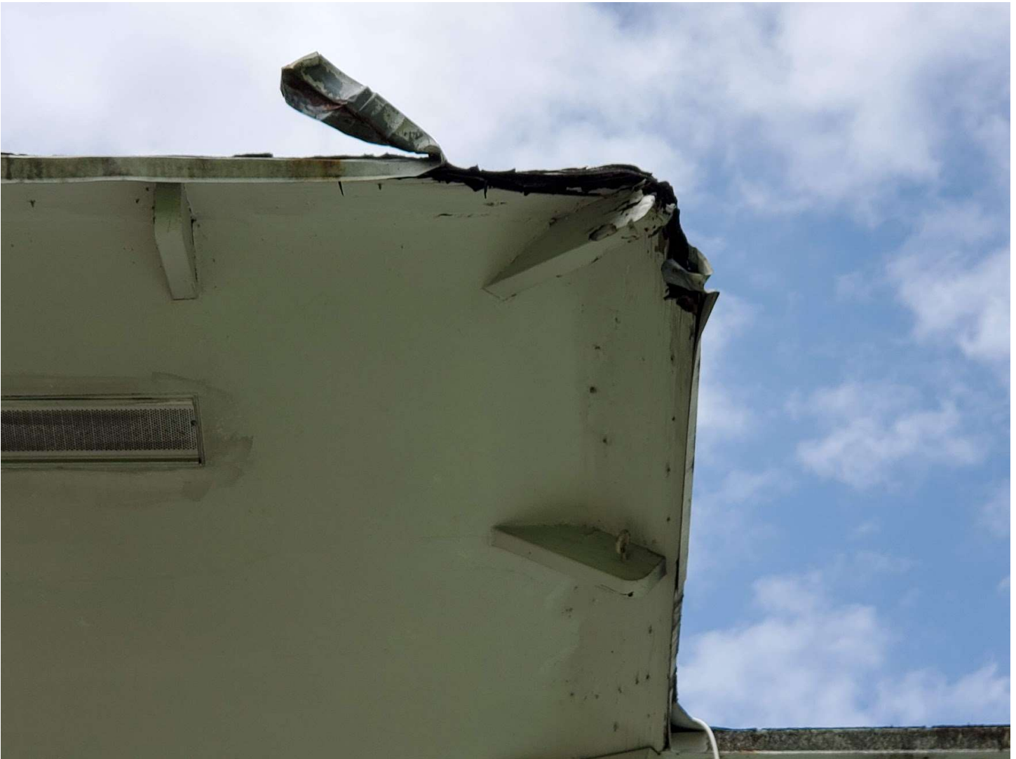
The roof of Building 7660; Example of damage to the eave of the mansard roof from trees adjacent to the building.
