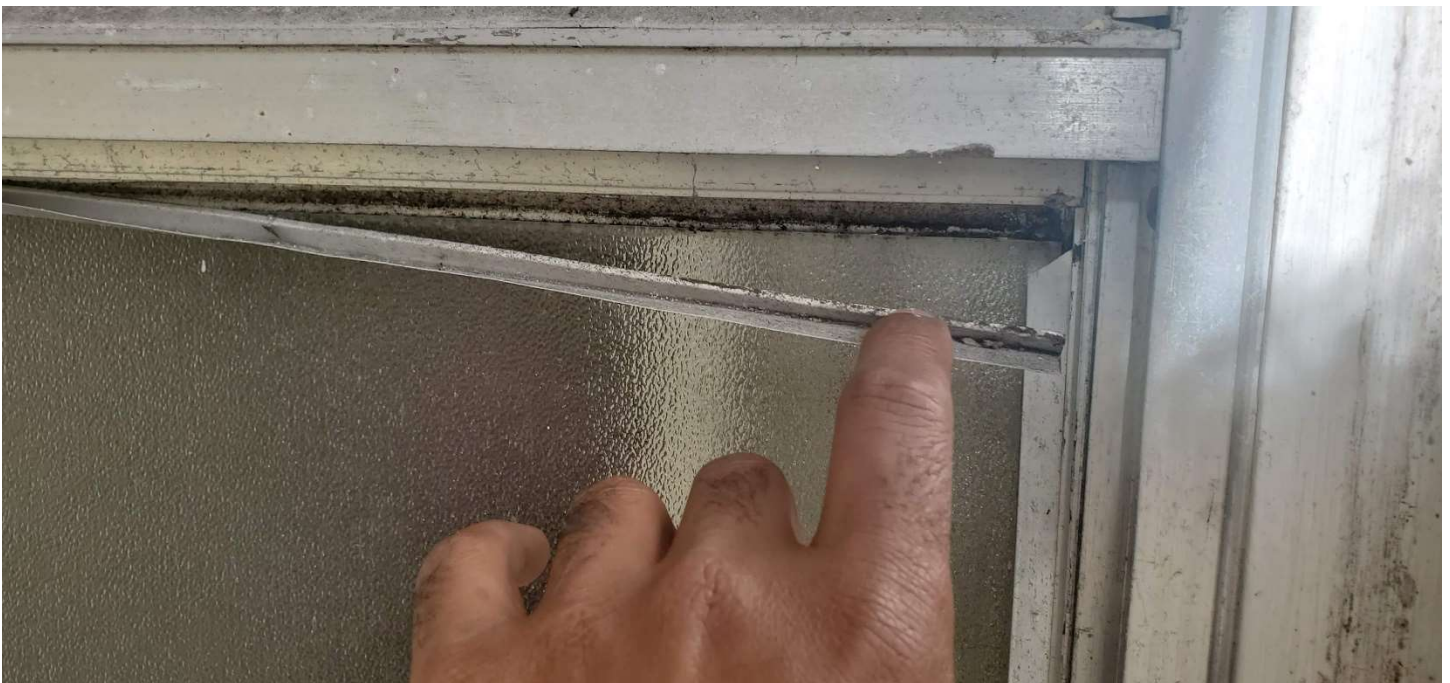
Single Hung Window A-7300-BF-12; Example of loose glazing in window sash/frame as a result of negative wind pressures from Hurricane Irma.
