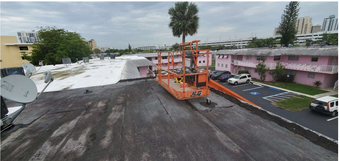
The roof of Building 7530; Example temporary roof repairs via a white sealant applied to the roof deck and temporary repairs to the delaminated build-up roof at the eaves.
