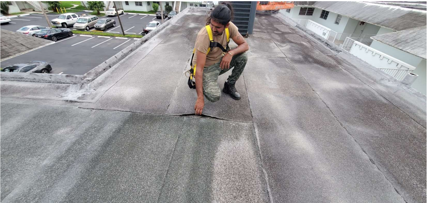
The roof of Building 7680 portrays an example of up-lift pressures causing delamination of the “modified bitumen membrane” top ply at the seams of the roof.
