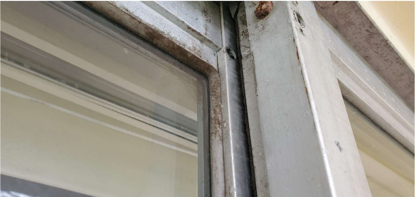
Close up of Sliding Glass Door A 7300-AB-02 example showing deformation to the door frame and failures of the door hardware causing binding during operation and out of the plane movement of the door panel as a result of winds from Hurricane Irma.
