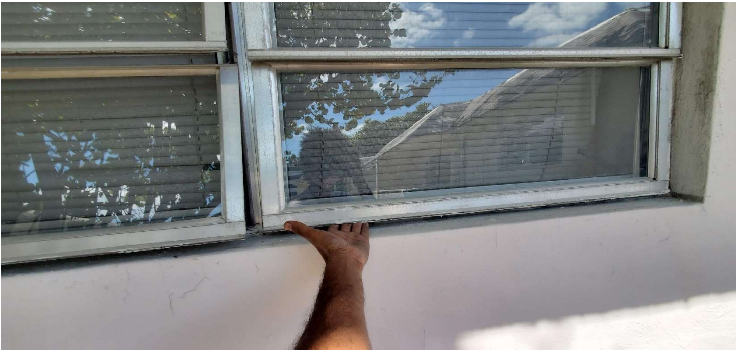
Awning Window C-7340-BR-02 example of winding/ locking mechanisms be affected by the wind pressures from Hurricane Irma. The window cannot be locked or completely closed and is not weather tight.
