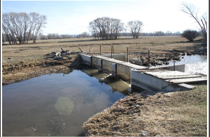
Feeder ditch diversion (CONSOLIDATED SLOUGH WEIR)
