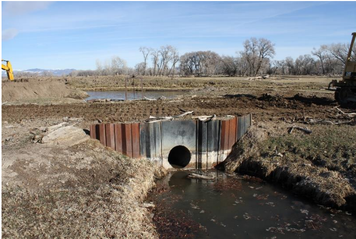
Trash rack at river headgate
