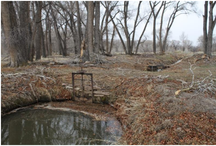
Headgate looking downstream
