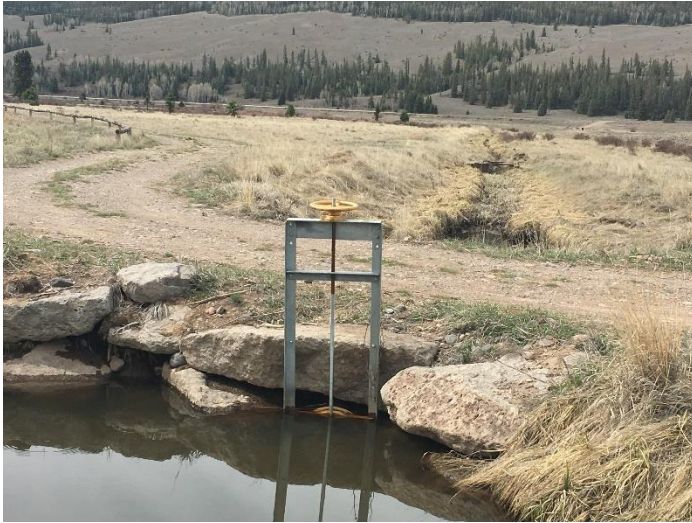
Headgate looking downstream
