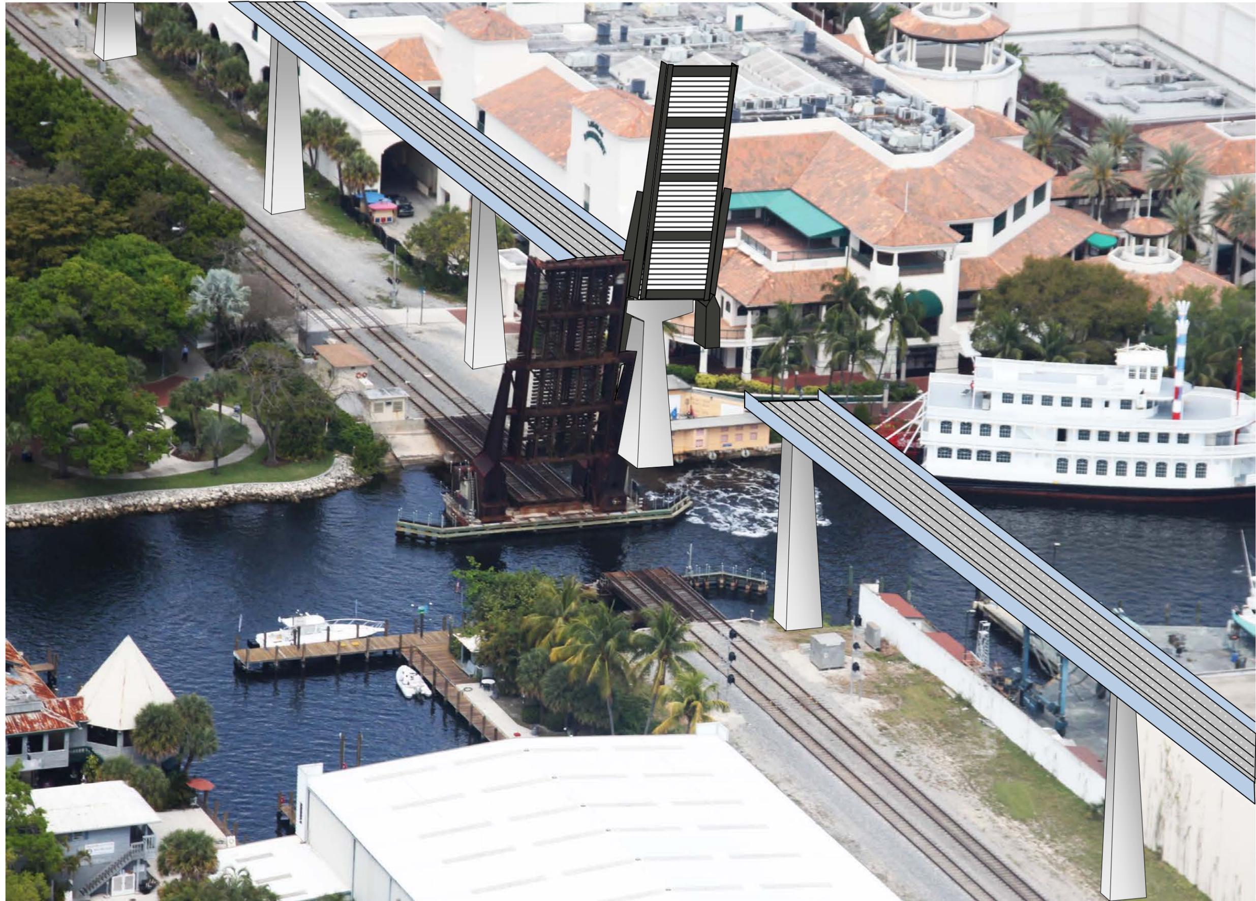
**CONCEPTUAL RENDERING OF HIGH LEVEL MOVABLE PASSENGER RAIL BRIDGE AND VIADUCT OVER THE NEW RIVER**
