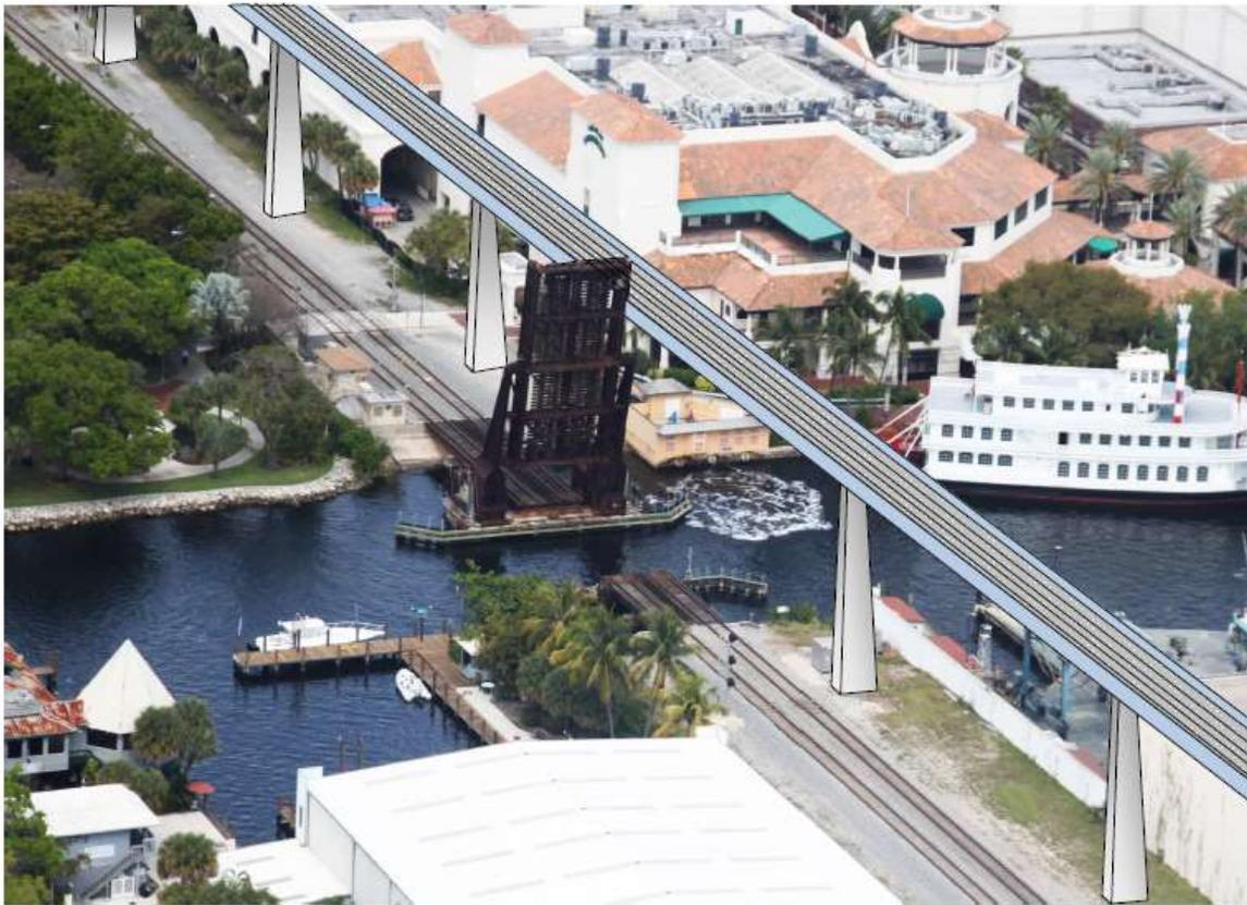
CONCEPTUAL RENDERING OF HIGH LEVEL FIXED PASSENGER RAIL VIADUCT OVER THE NEW RIVER
