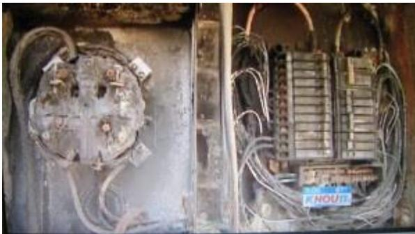
In Chicago, smart meters were identified as being the cause of several fires in suburban homes in which Commonwealth Edison installed the devices. Other smart meters were found to overheat severely while in service.
