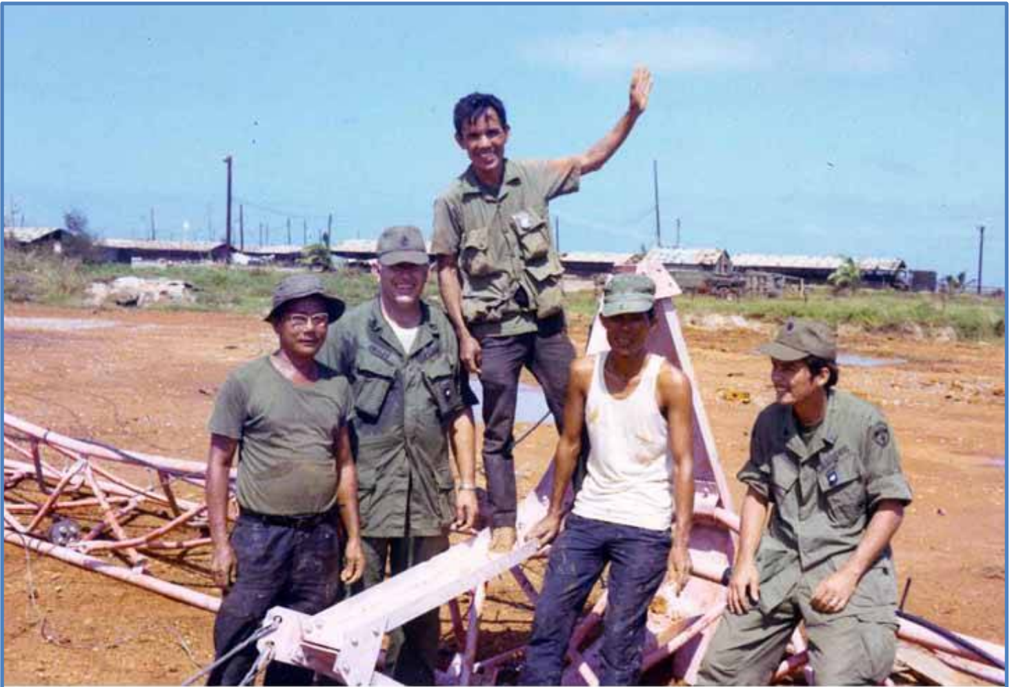
With some of the AFVN "local hire" tower crew taking down the Chu Lai tower.
