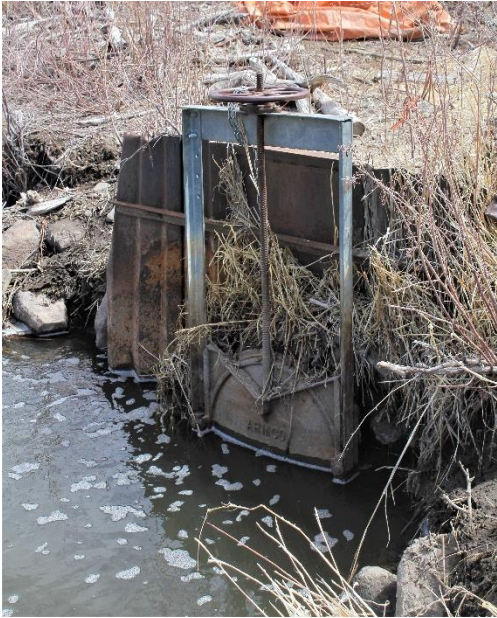
Headgate looking downstream
