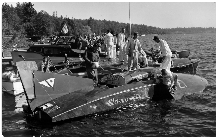
Slo-mo-shun IV during early tests in 1952. A trim tab with a square top has been added to the tail.
