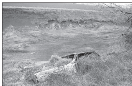
Source: GAO. Abandoned Car in Canal
