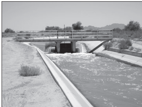
Source: GAO. Concrete-lined Irrigation Canal
