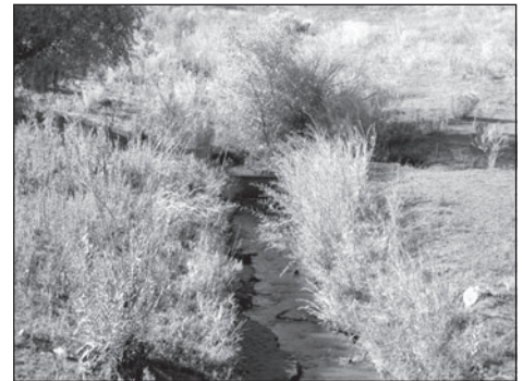
Overgrown Vegetation in Irrigation Ditch
