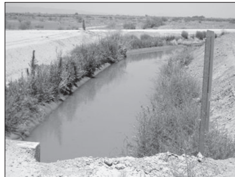
Canal with Vegetation Growth
