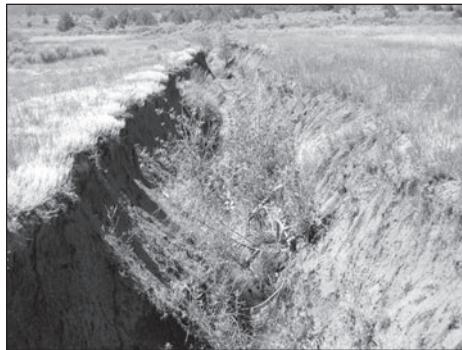
Irrigation Ditch in Need of Reshaping
