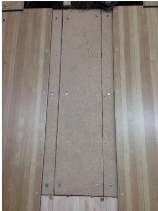
I secured both sides of the keyway cut with the 4" #16 screws.
