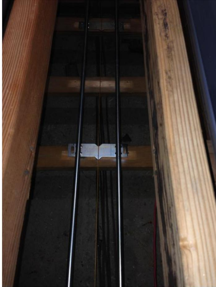
We connected all of the track sections and ran a string from the centerline of the downsweep to the centerline of the powerlift up front, and secured the new track under the stringline.
