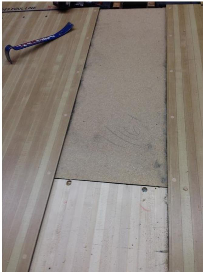
So I cut them a keyway and secured the replaced underlayment outside the cut.
