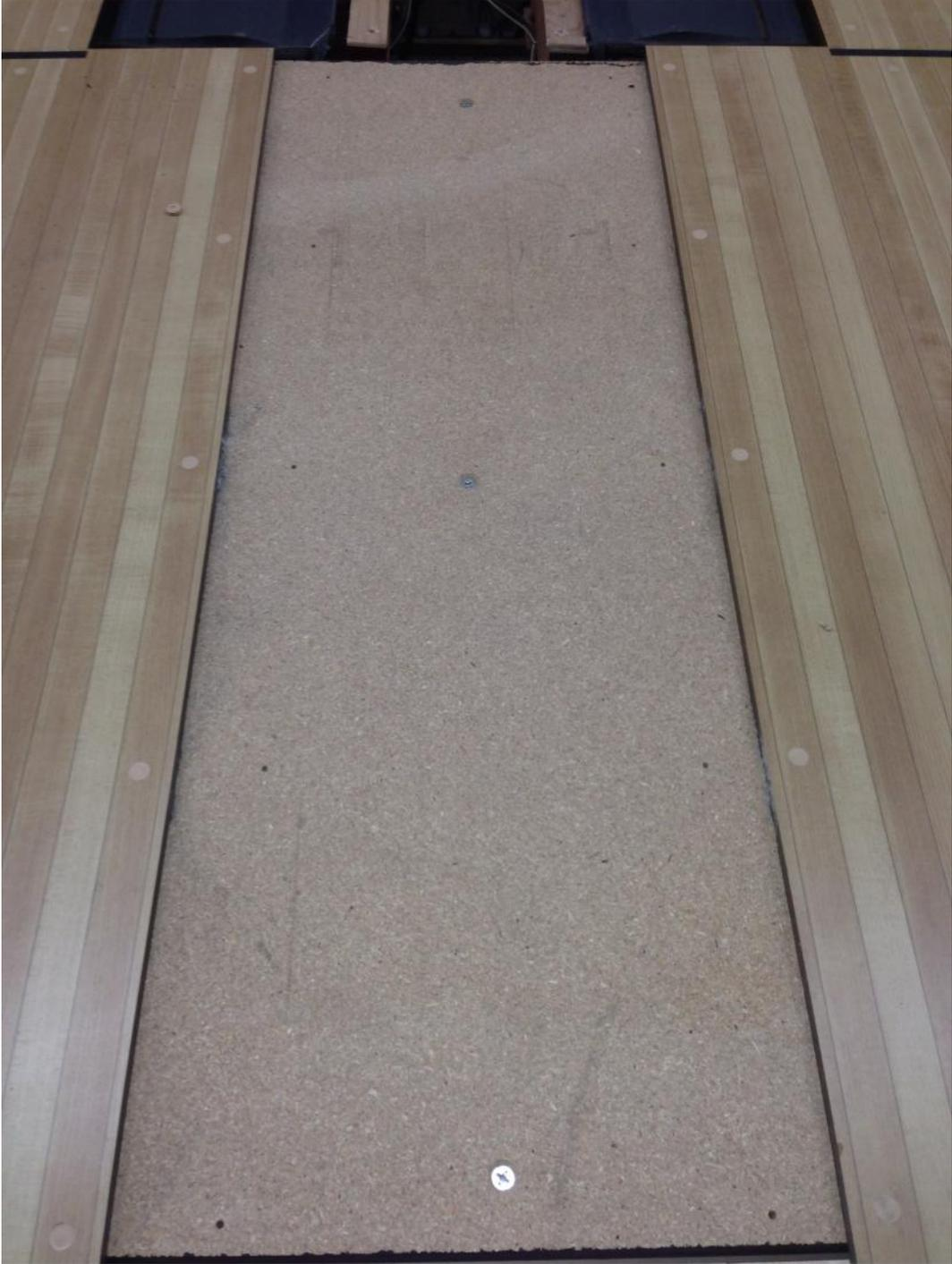
These screws were so long that they were in the ball's path as the balls returned. All of the screws were badly bent and a pile of ball chips was in the underlane.
