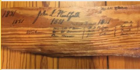
This photo is a builder's board recovered from the Center Hill house in eastern Orange County, dating to the early 1850s. This artifact was found after removing finish lathe and plaster over a first floor wall cavity. The builder's board dates to 1851 and clearly displays the name of the master carpenter and his work crew.
