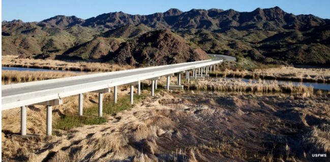
BILL WILLIAMS RIVER BRIDGE, HIGHWAY 95
