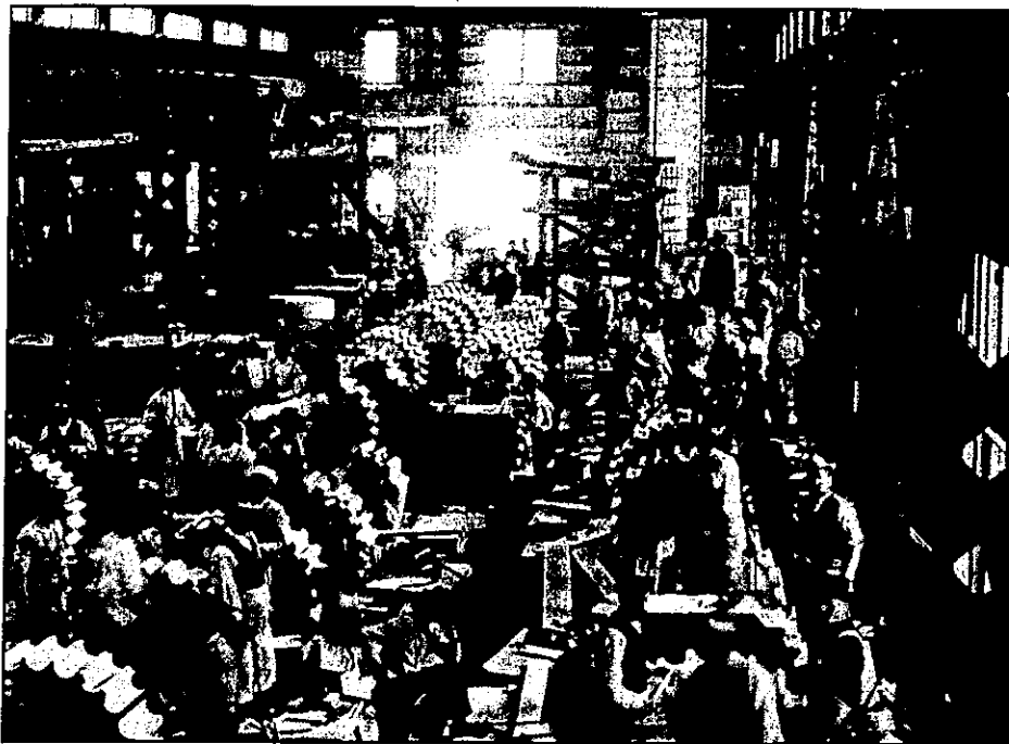
Figure 23. An impressive 1912 west-looking view of Shop 3, also known as the monumental shop, where column drums were prepared for large projects (Frank Gertif collection, from McCollum 1993:94).
