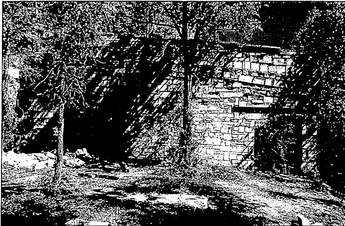
Figure 45. Firewall No. 2 between Mill B and the Coping Shop is at its original height and appears stable. Photo looking east.
