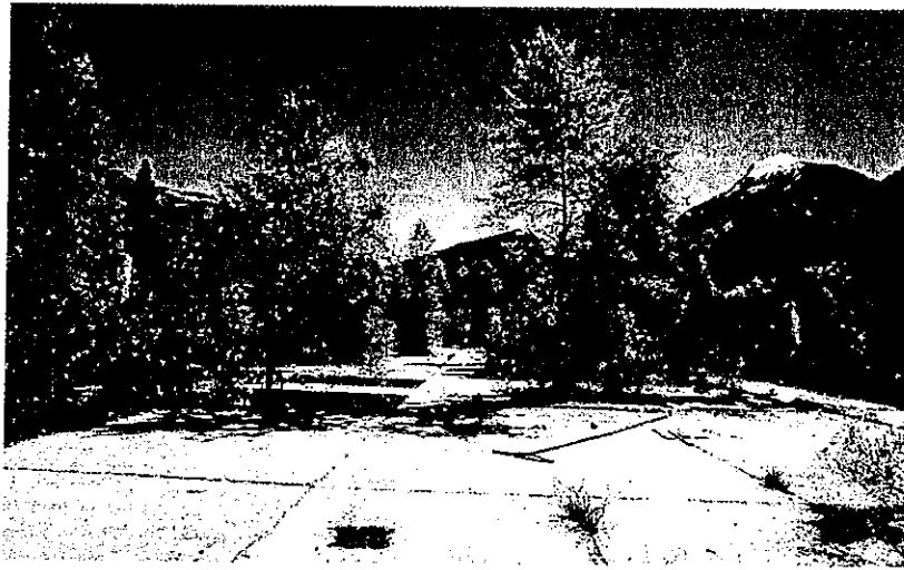
Figure 7. Overview of Shop 2, looking west. Concrete slab floor is intact and boundaries are well-defined.
