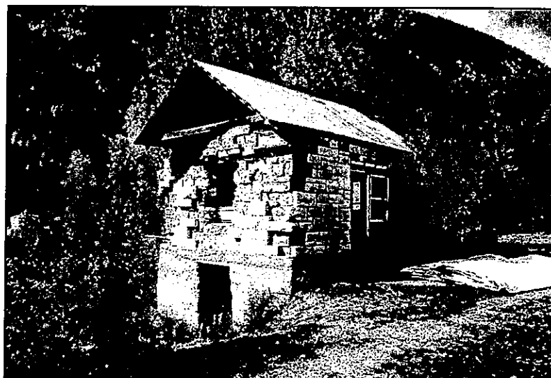
Figure 29. The Document Storage Vault is one of two structures that remain standing today. Much of the marble facing has been robbed, and the window/doorway is not original. The gable roof was installed to protect the building from weathering. Photo looking south-southeast.
