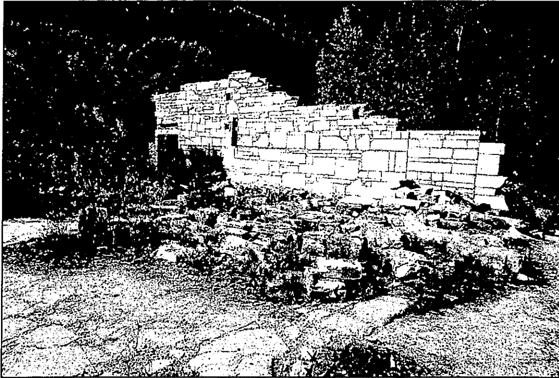
Figure 44. Although partially collapsed, Firewall No. 1 between Shop 2 and Mill B appears stable. Photo looking south-southwest.
