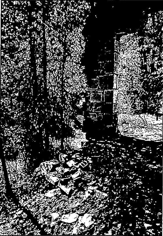
Figure 46. The stability of the doorway in the Firewall No. 2 is questionable due to foundation alteration and erosion. Photo looking west-southwest.
