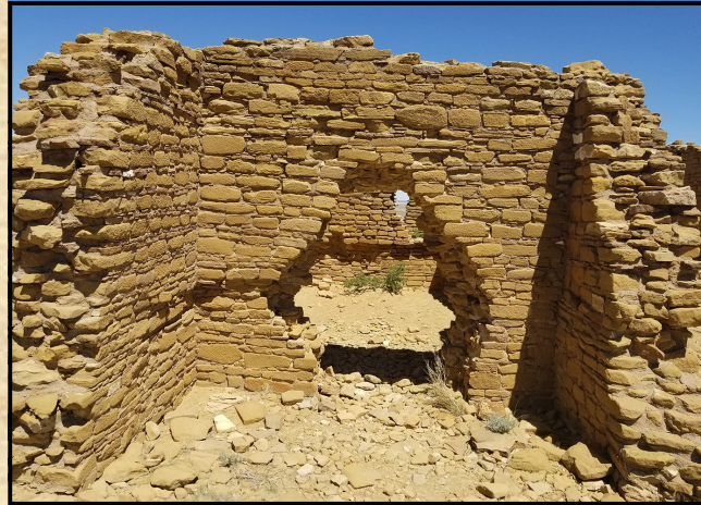
Doorway passage in Pueblo Bonito
