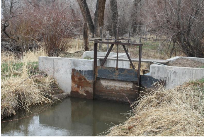
Headgate looking downstream
