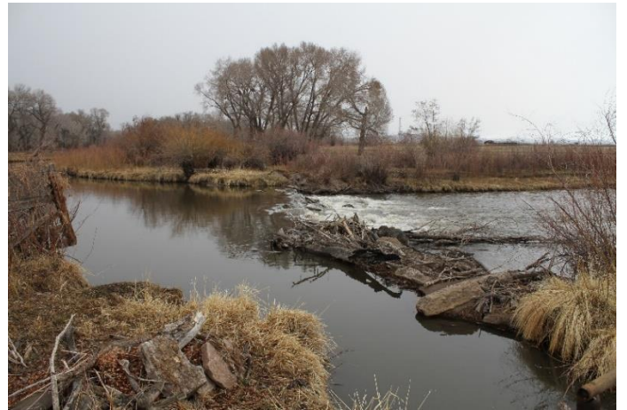
Diversion dam and feeder ditch
