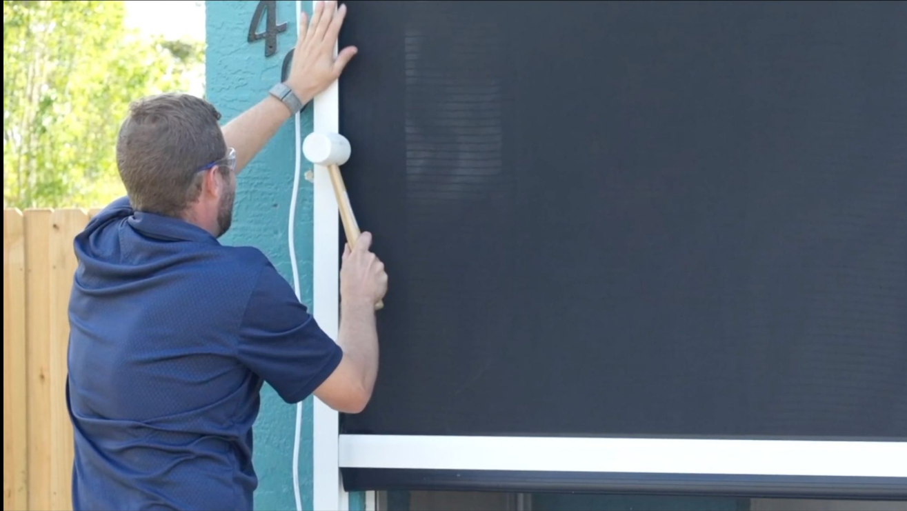
Attach track covers using rubber mallet
