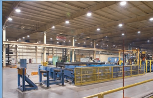
Duquesne Electric 1000 Watt Existing – Before. ← → Duquesne Electric – After T9-630 Watt MH-XL-Direct.
