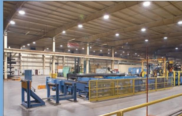
Warehouse Replaced 1000 Watt with T9-315 Watt MH-XL-Direct.
