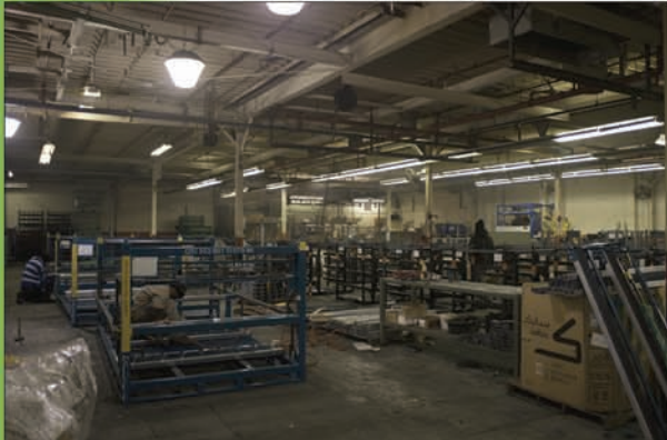
Duquesne Electric 1000 Watt Existing – Before. ← → Duquesne Electric – After T9-630 Watt MH-XL-Direct.
