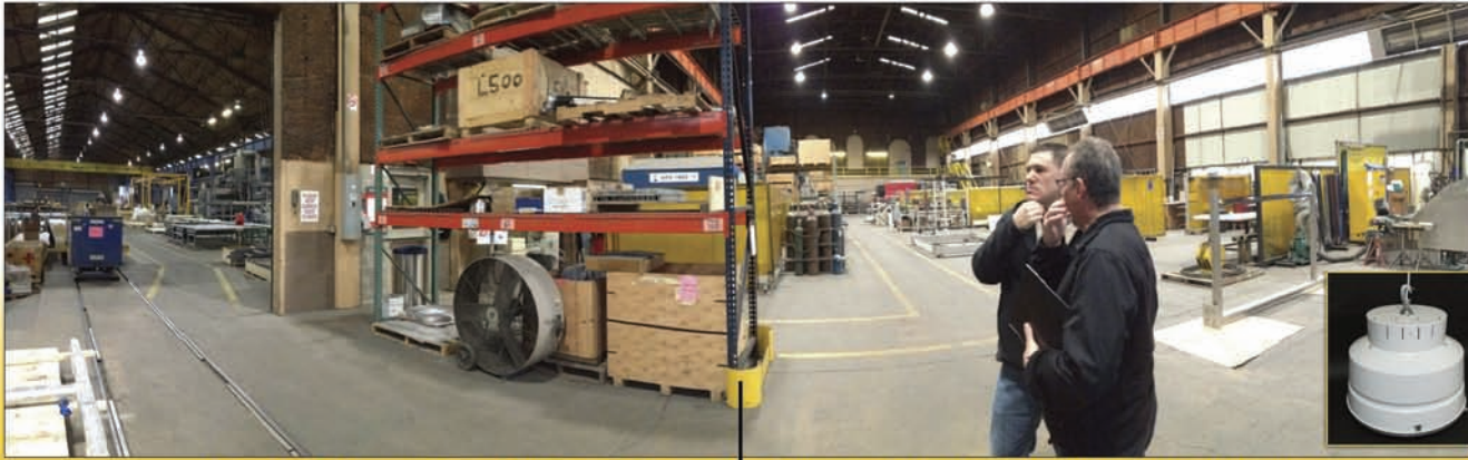
Duquesne Electric 1000 Watt Existing – Before. ← → Duquesne Electric – After T9-630 Watt MH-XL-Direct.
