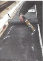
Fuse adhesive is the recommended adhesive for applying the mats in cold temperatures (<40°F). Apply along outer edges of the mat with a single line down the center. If mats need to be removed from the roof at any point, turn the mat on, let it warm up, then slowly and gently pull the mat up.
