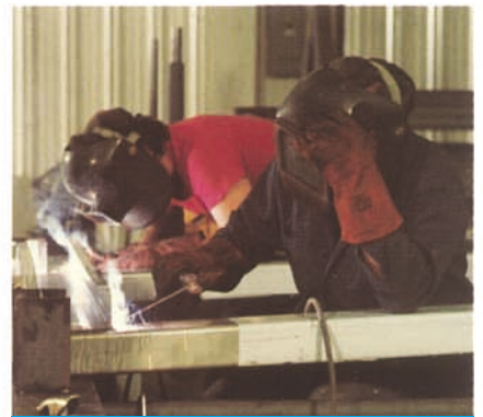
Welding vertical support structures
