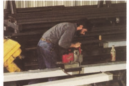
Fabricating stainless steel supports
