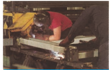
Fabricating vertical members in welding jig
