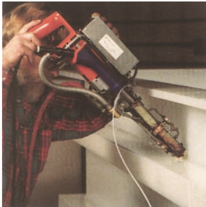
Extrusion welding process
