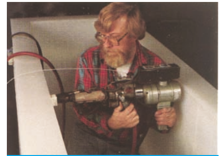
Technician with extrusion welder fabricating tank flange
