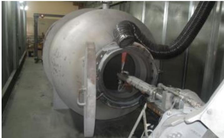
Application of Hastelloy C coating inside the sulfur removal plant vessel
