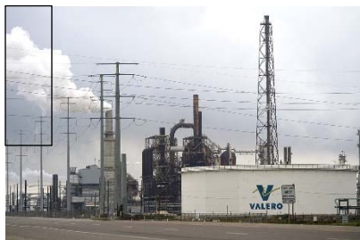
An oil refinery in Texas. | David J. Phillip/AP Photo
