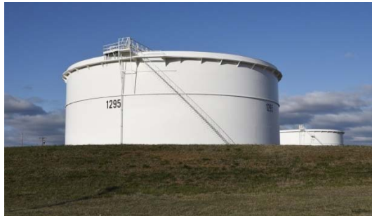
Crude oil storage tanks at a tank farm in Cushing, Okla., in 2016.
