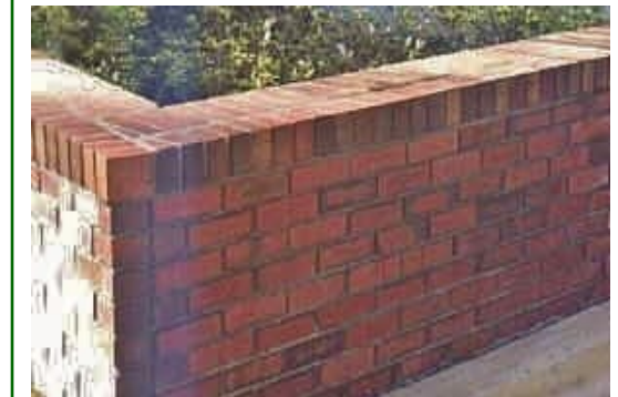
Before & After Efflorescence Removal
