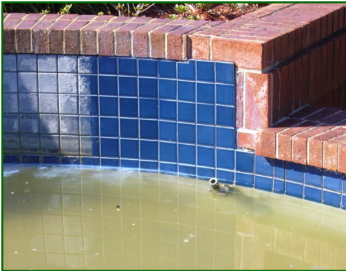
Tile and Grout Restoration
