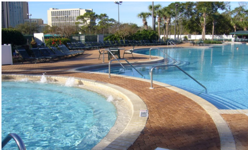
Before & After Paver Stone Restoration
