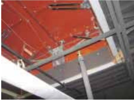
Installing a fire sprinkler below a vent is a common mistake that makes it likely that one or both will not function as intended. Also, the manual release, suitable for use on a 20' warehouse roof, is frequently inaccessible to occupants on a stage.
