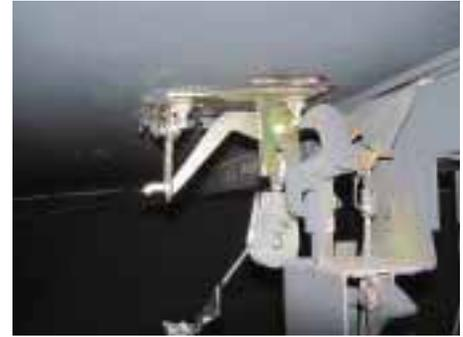
Computer modeling shows that a fusible link mounted on the vent will not open until well after the audience has left the auditorium. This vent has been modified for stage floor operation, which has nullified the conditions of it being labeled.
