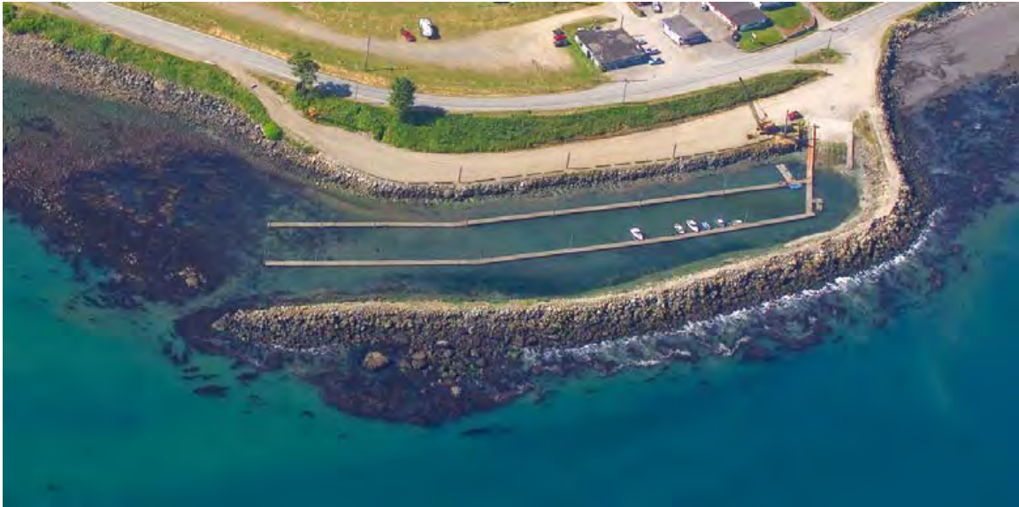
Figure 4. Example of artificial shoreline, this feature between Clallam Bay and Sekiu (source: DOE 2006).
