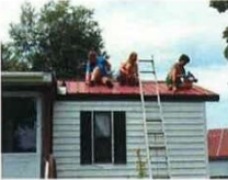
Removing nails from roof, replacing with screws
