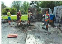
Cleaning up debris from building fire
