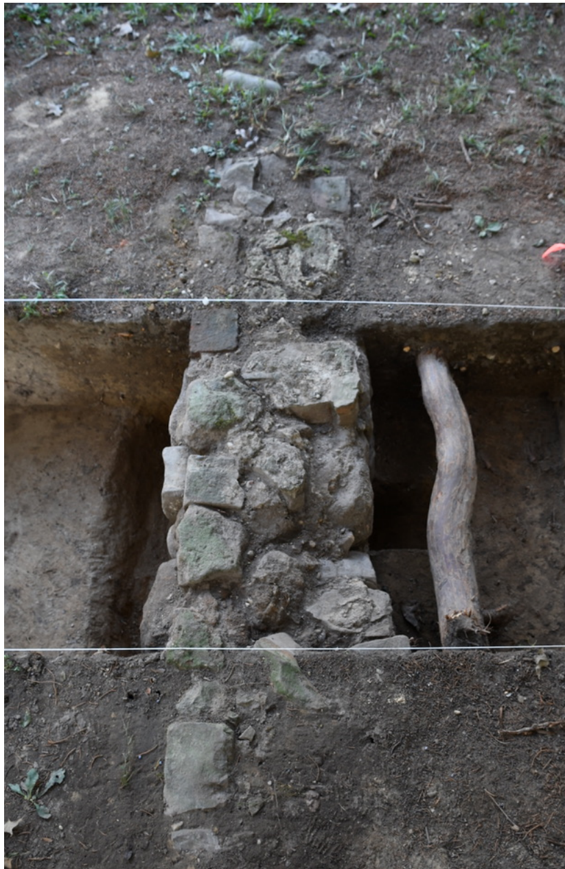
Figure 20: Top of Feature 1 wall foundation; looking east.
