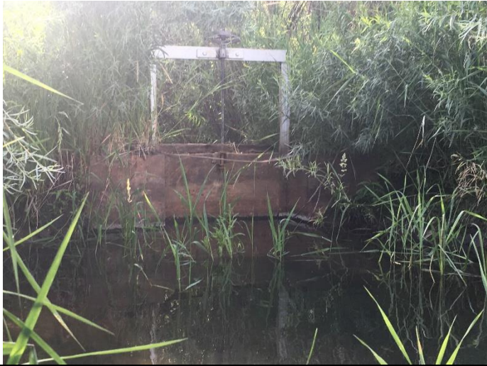
Headgate looking downstream
