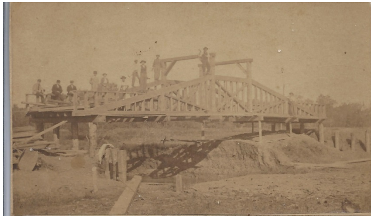
A Bridge Under Construction
