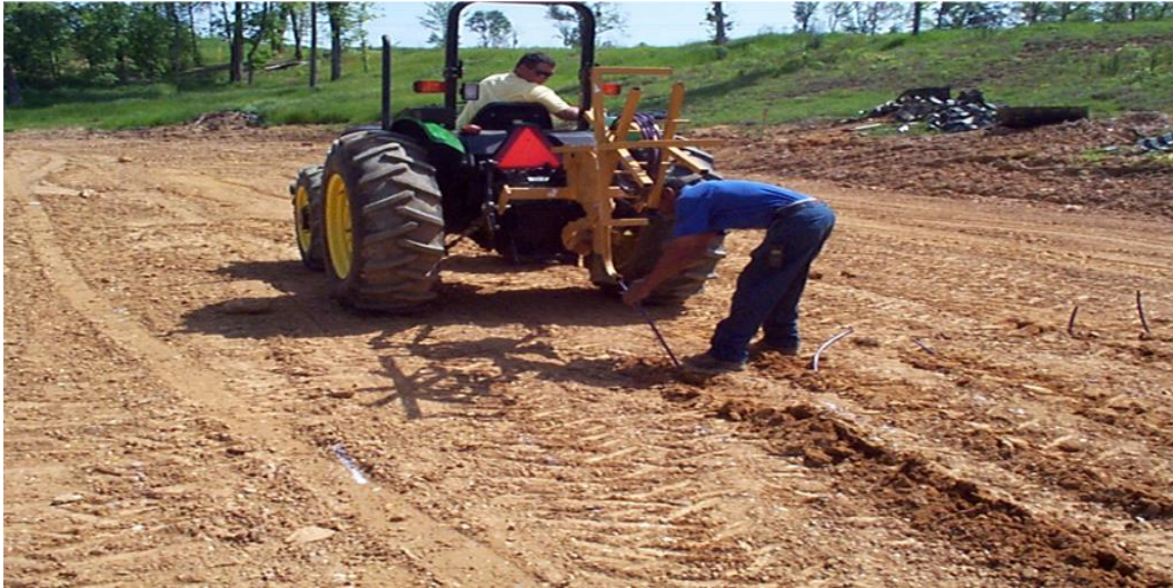
Dripline Insertion by Trenching with Single-Reel. Multiple Reels Also Possible
