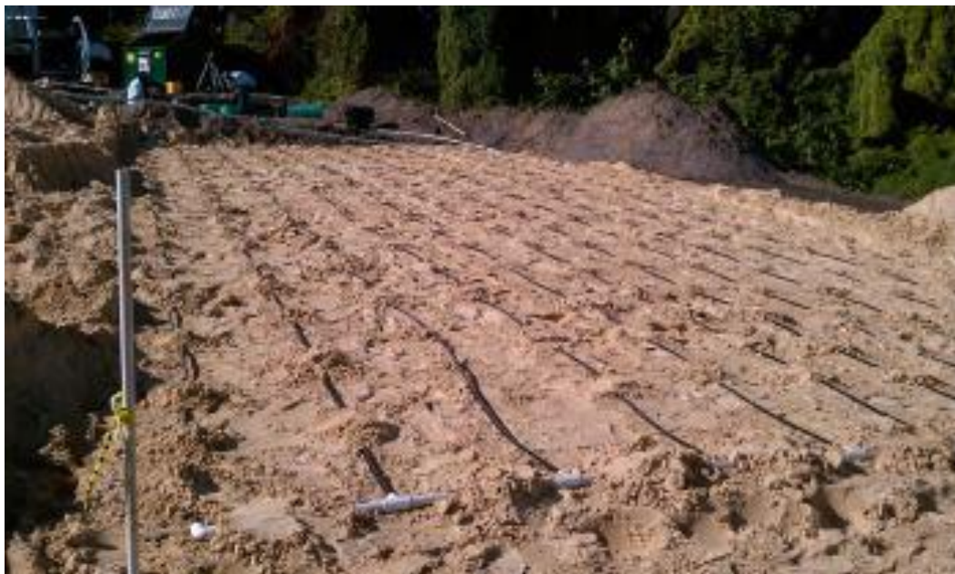
Dripfield Installed Without Trenching. Cover with 6 to 9 inches of Soil & Vegetate.
