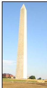
Washington Monument Renovation
