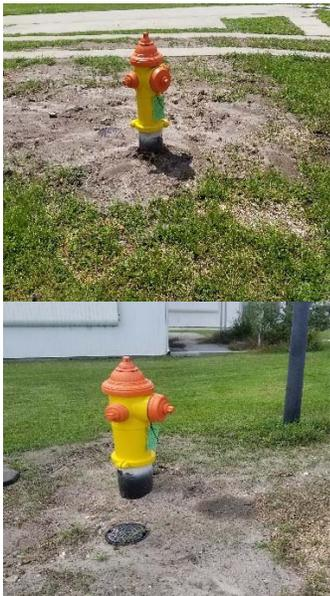
Two new Hydrants were installed this summer, one on 21-16 and another on 11-18. these new hydrants will help our Fire Dept. In case of fires, with the smaller truck it has less capacity
