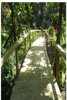
To the left is a picture of the new Boardwalk that The Maintenance Dept. constructed this summer (70ft long with safety railing) also several of the deckboards were replaced on the old boardwalk
