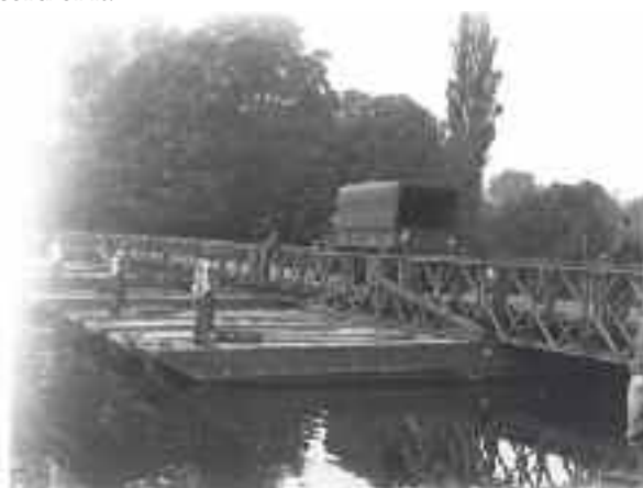
Bailey Bridge building at Pangbourne. (Photo courtesy of the Heritage Group.)
