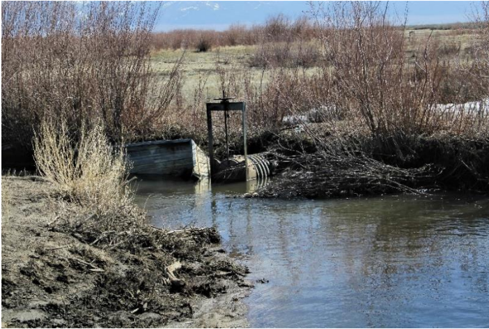
Headgate looking downstream
