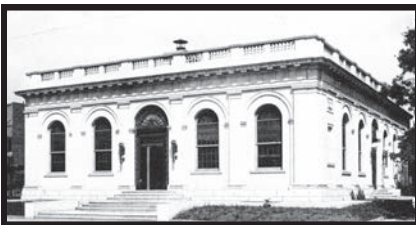
Federal Post Office Building circa 1913
