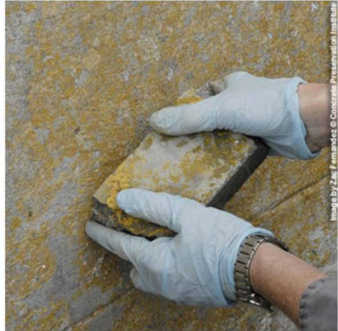
A variety of methods are used to replicate the appearance of the existing concrete, some of which has more than 100 years of patina and color. Image by Zac Fernandez © Concrete Preservation Institute
